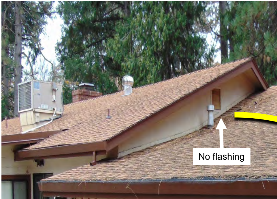
Item 3.1 Roof Assembly Details (Flashing) – Flashing to protect against ignition by combustible debris and embers.
