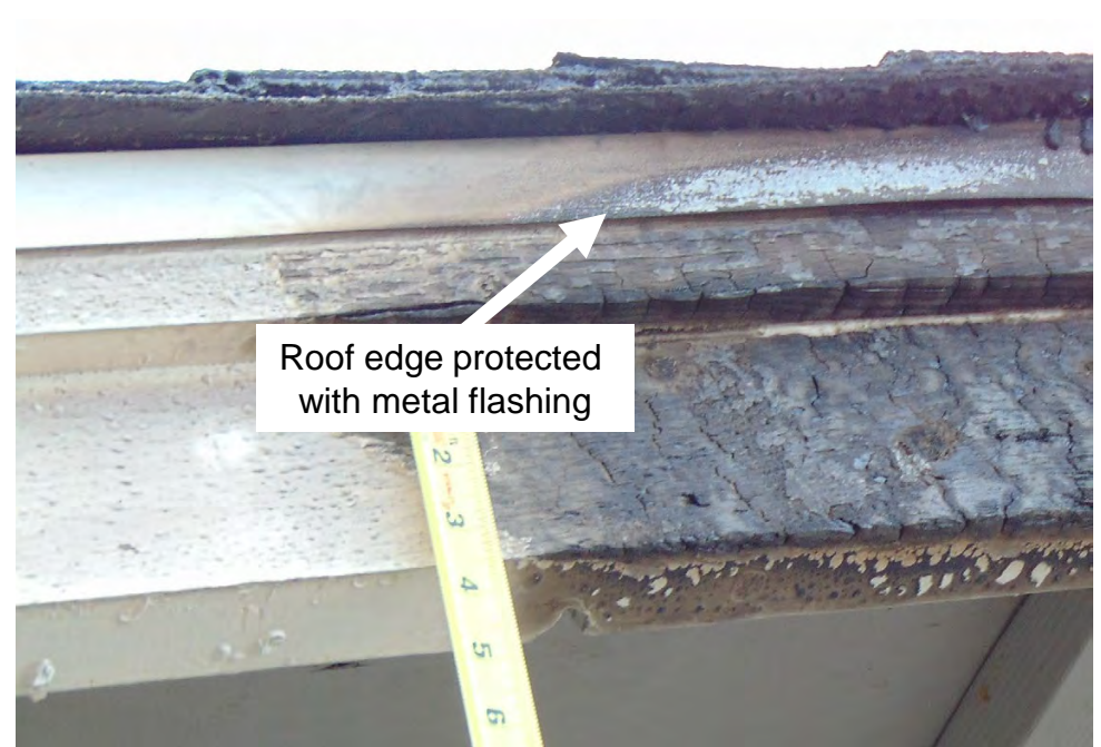
Item 7 Roof Covering with Openings – Roof deck exposed when roof covering material or flashing does not extend past the roof deck or is not present.
