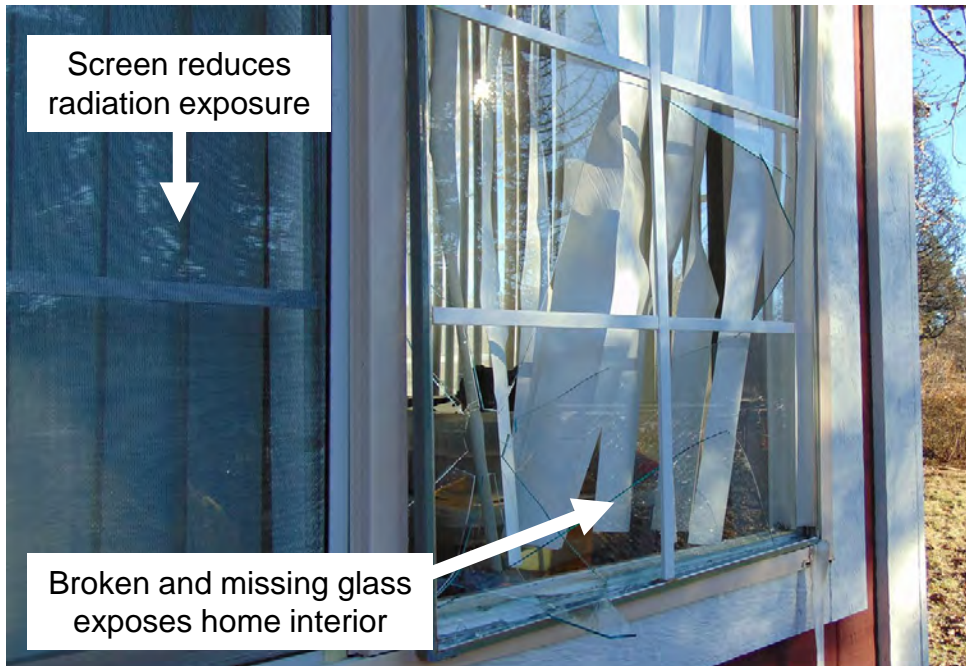
Item 23 Window (Double Pane) – Double pane provides protection against radiation and ember intrusion.
