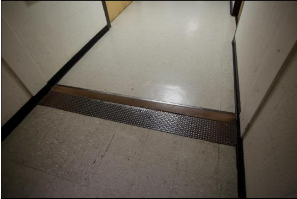
Photo C-137. Typical Expansion Joint Cover
