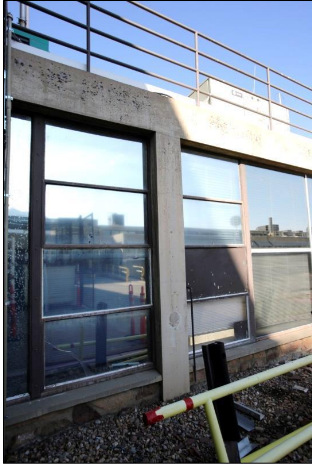
Photo C-19. Original Windows on South Elevation (view north)
