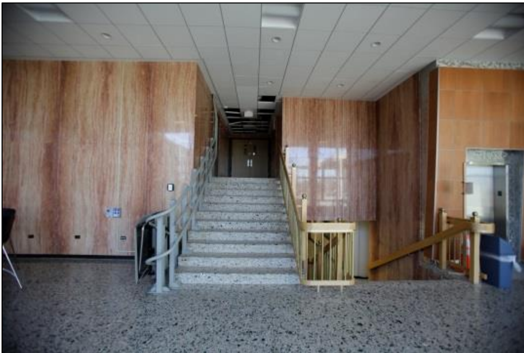
Photo C-98. Lobby Stairs to Levels 1 and 2 of the Spine (view southwest); the handrails were originally 1.5-inch steel pipe
