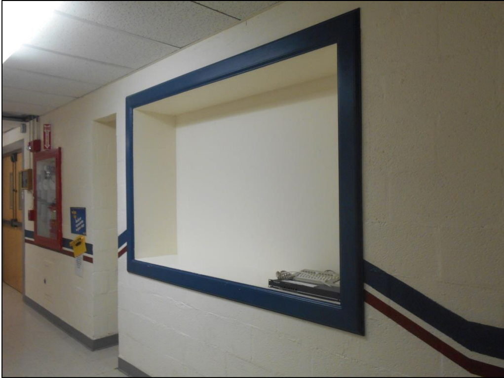
Photo C-133. Infilled Atomic Clock Viewing Window
