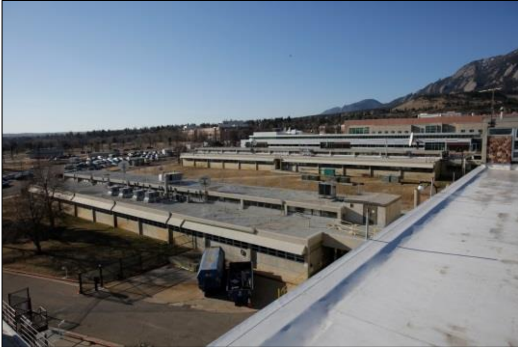
Photo C-55. View of Roof of Wing 2 from the Roof of the Spine (view south)
