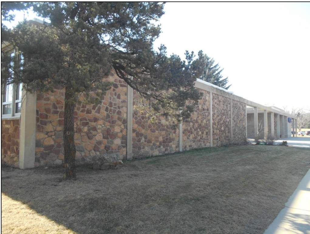
Photo C-14. North Elevation of Library (view west)
