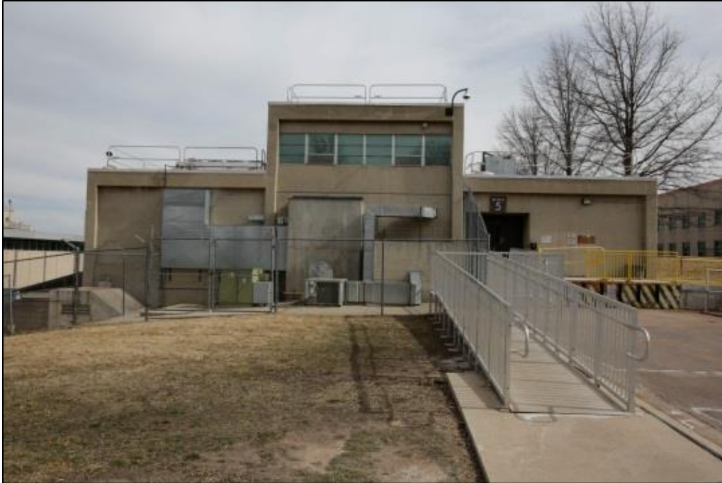
Photo C-69. West Elevation of Wing 5 (view southeast)
