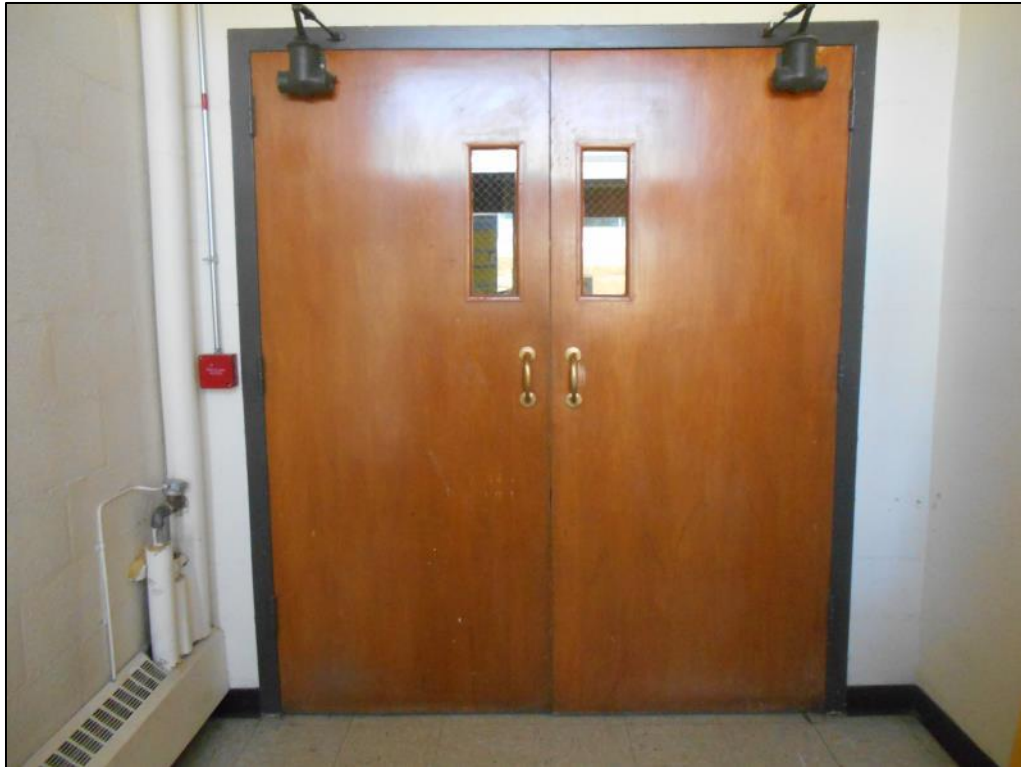
Photo C-141. Original Doors in Wing 1
