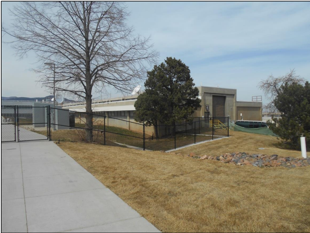
Photo C-58. South and East Elevations of Wing 4 (view north)
