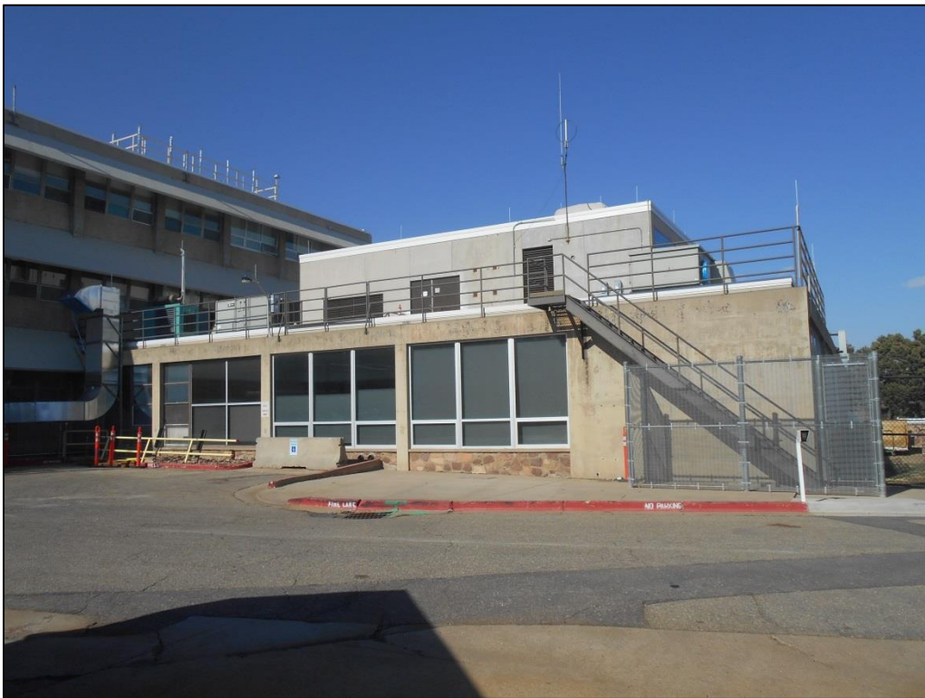
Photo C-18. South Elevation of Library (view north)
