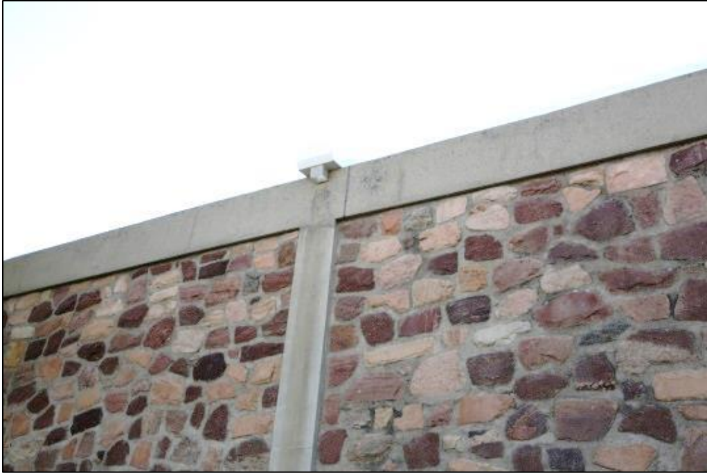
Photo C-15. Detail of North Elevation of Library (view southwest)
