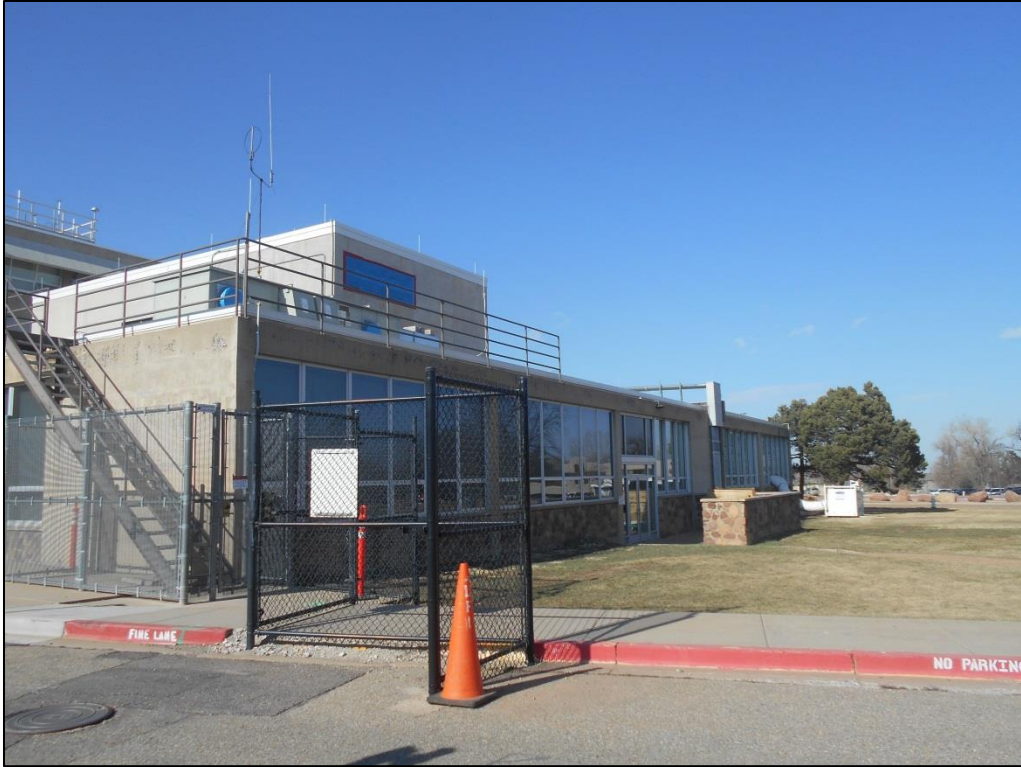
Photo C-17. East Elevation of Library (view north)
