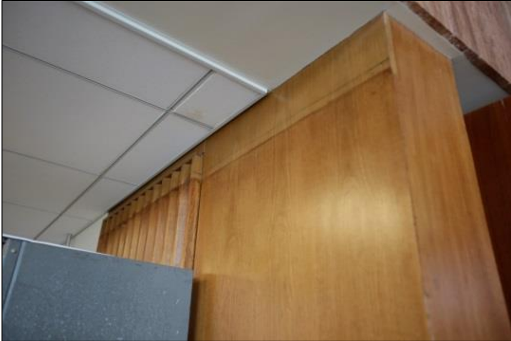
Photo C-111. Wood Wall Paneling in the Reception Area
