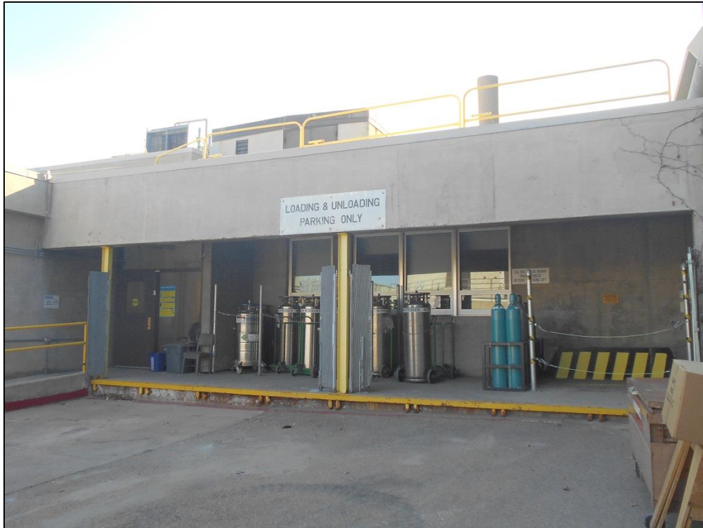
Photo C-53. Loading Dock on the North Elevation of the Hyphen between the Spine and Wing 2 (view southwest)
