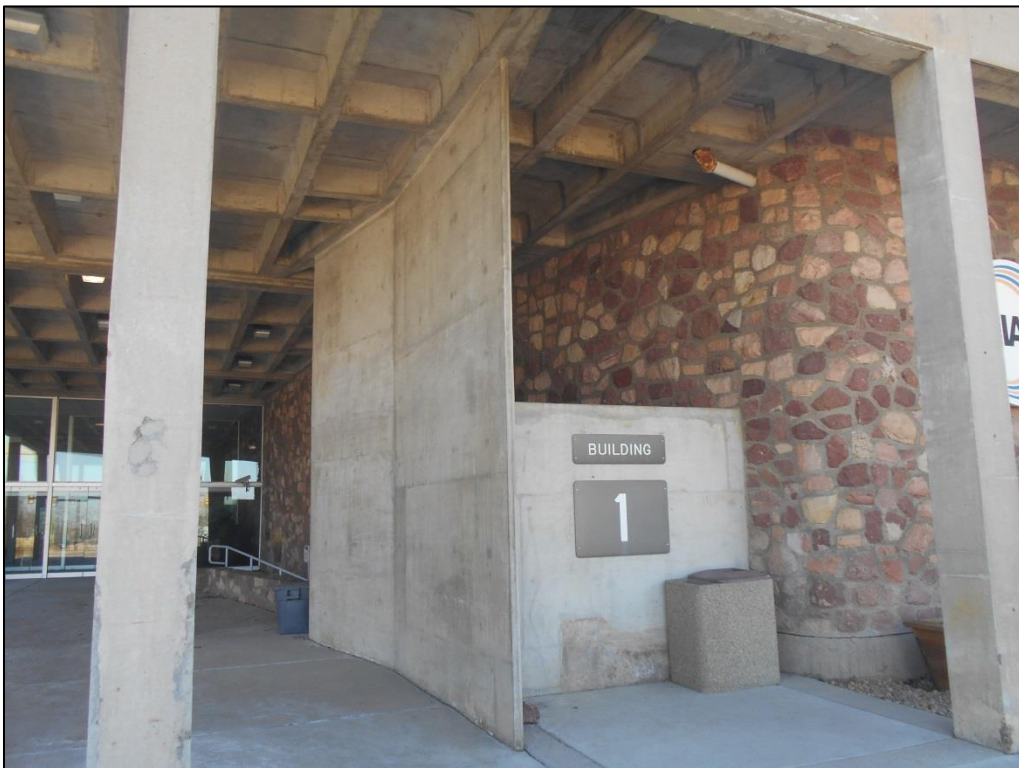
Figure C-8. Northeast Corner of Auditorium (view southwest)
