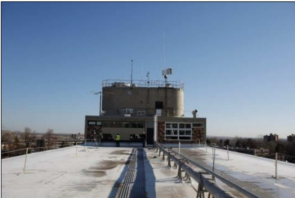
Photo C-30. South Elevation of the Rooftop Penthouse (view northeast)
