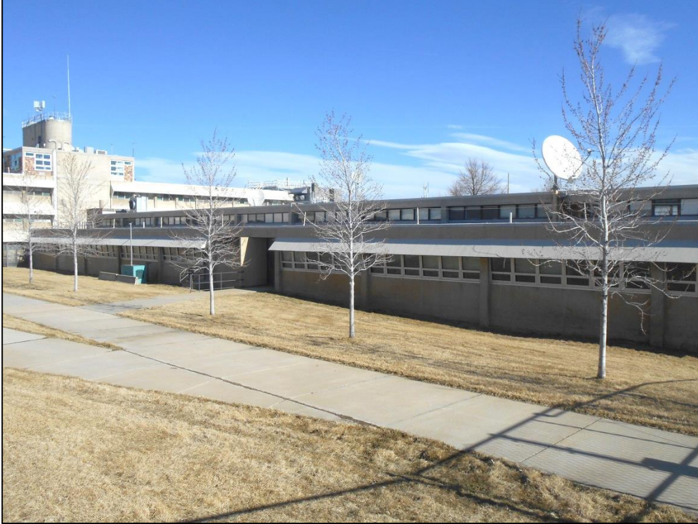
Photo C-51. South Elevation of Wing 2 (view north)
