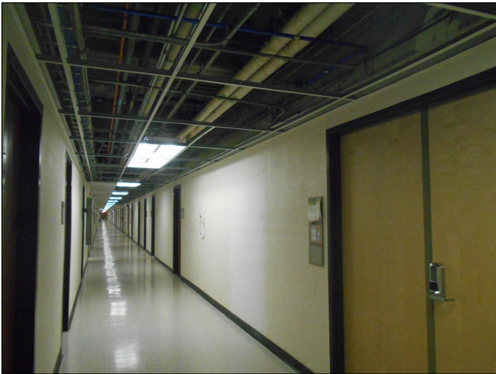
Photo C-136. Level 3 Spine Corridor (view southwest)
