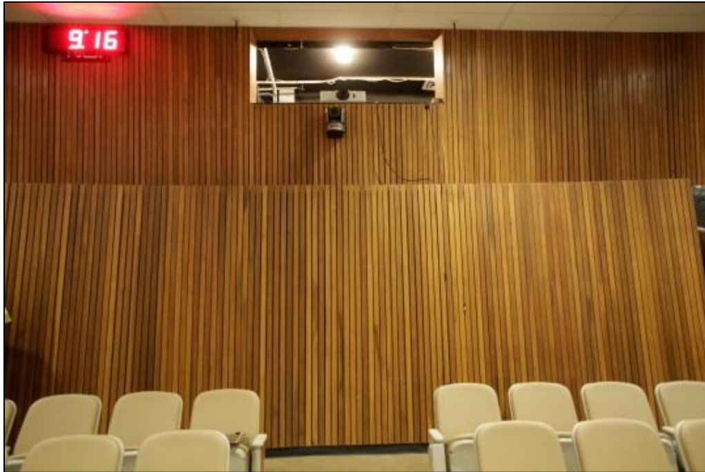
Photo C-75. South Wall of Auditorium (view southwest)
