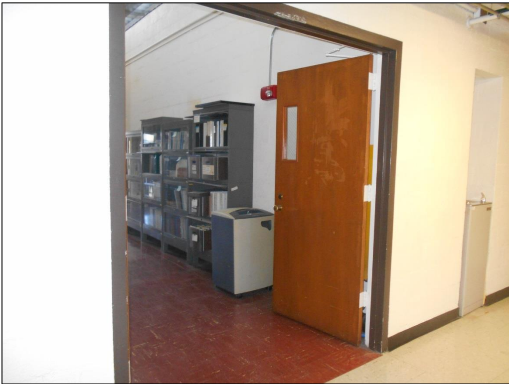
Photo C-146. Original Door and Asphalt Tile Flooring in Wing 4
