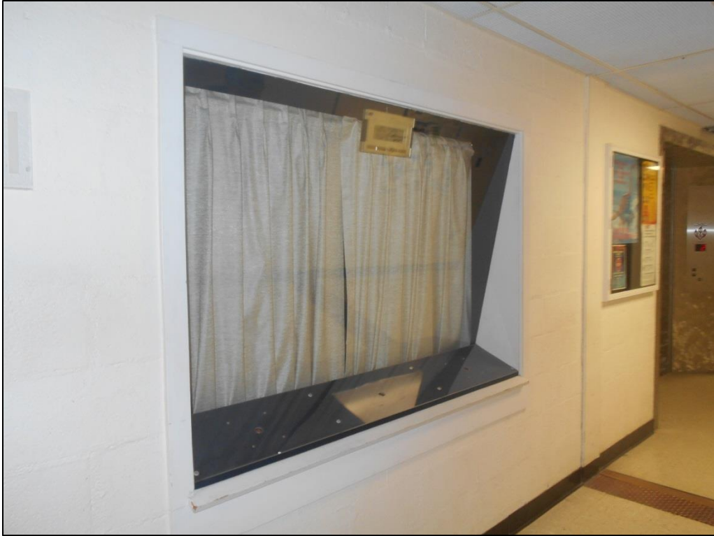
Photo C-139. Curtained Viewing Window in Level 4 of the Spine.
