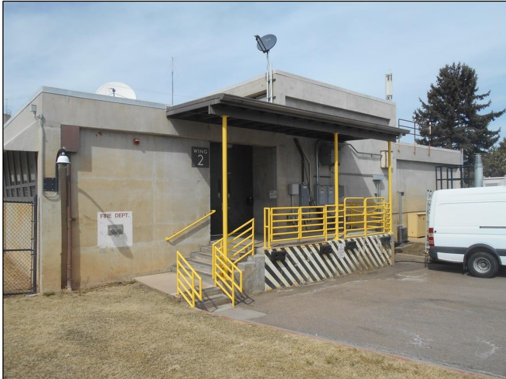
Photo C-54. Loading Dock on the East Elevation of Wing 2 (view north); the cantilevered shade and the metal pipe railings are not historic features of this elevation
