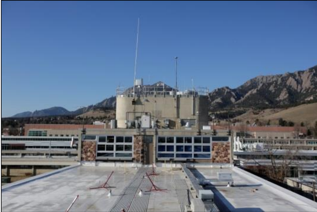
Photo C-31. North Elevation of the Rooftop Penthouse (view southwest)
