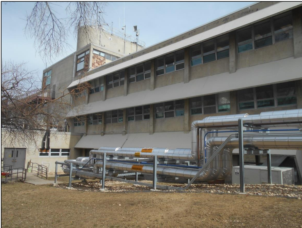
Photo C-24. West Elevation of Spine (view northeast)
