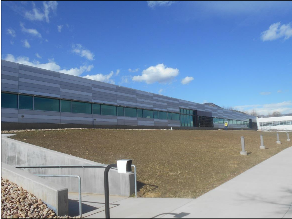
Photo C-71. East Elevation of Wing 6 (view west)
