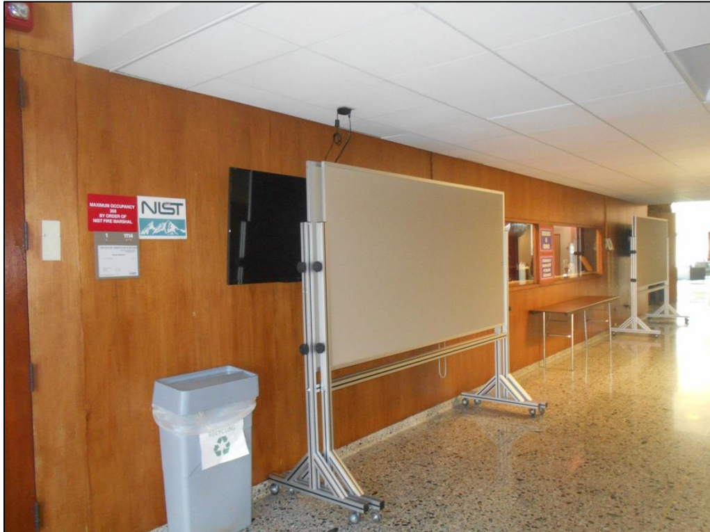
Photo C-96. North Wall of the Foyer between the Entrances to the Auditorium (view east)
