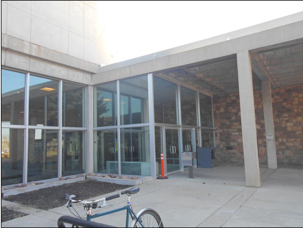
Photo C-21. Vestibule and Main Entrance to Lobby (view west)
