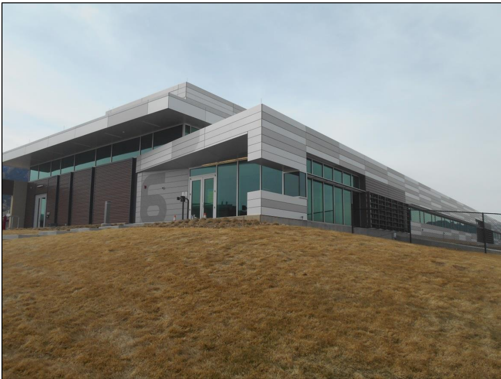
Photo C-70. South and East Elevations of Wing 6 (view west)
