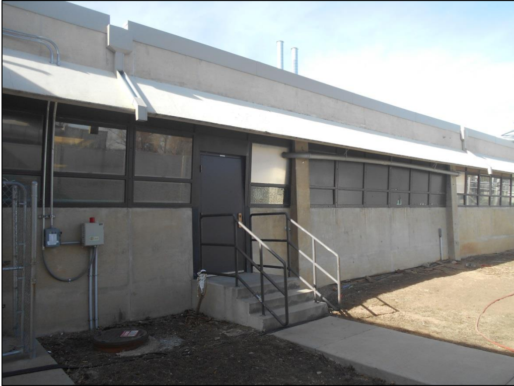
Photo C-39. Original Door on North Elevation of Wing 1 (view southwest)
