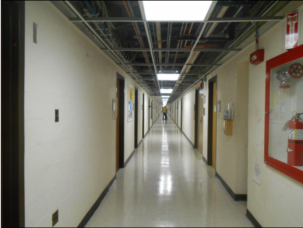
Photo C-135. Level 3 Spine Corridor (view northeast)
