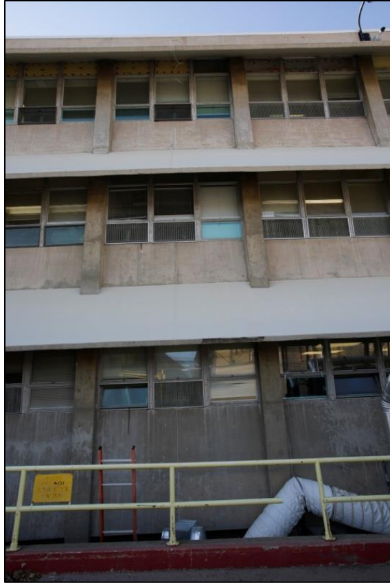
Photo C-25. East Elevation of Spine (view northwest)
