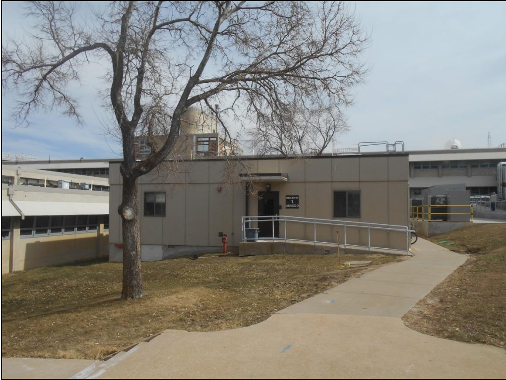
Photo C-43. Annex D South of Wing 1 (view southeast)
