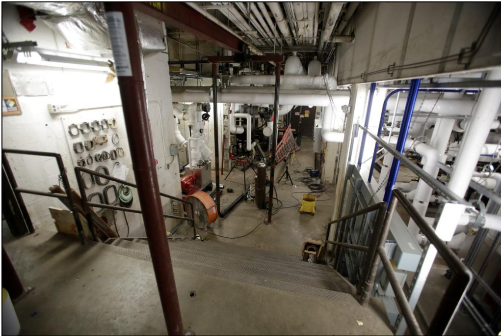
Photo C-122. Boiler Room Area in Level 1 of Spine (view southwest)
