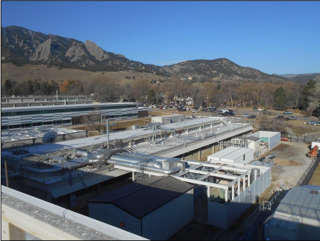
Photo C-44. Rooftop of Wing 1 and Annexes E and F (view west)
