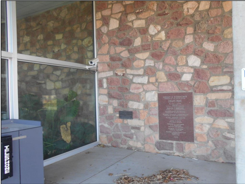
Figure C-10. Cornerstone in East Wall of the Auditorium (view west)
