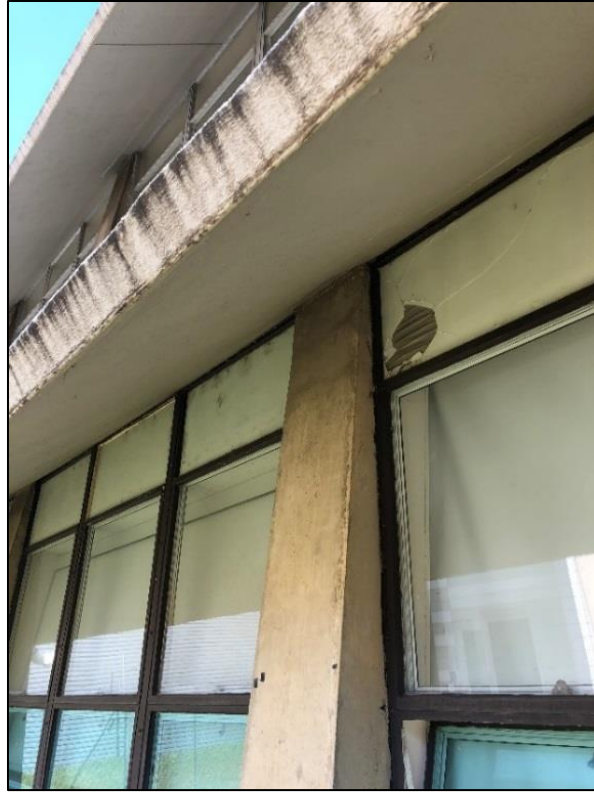
Photo C-157. Sunshade Staining
