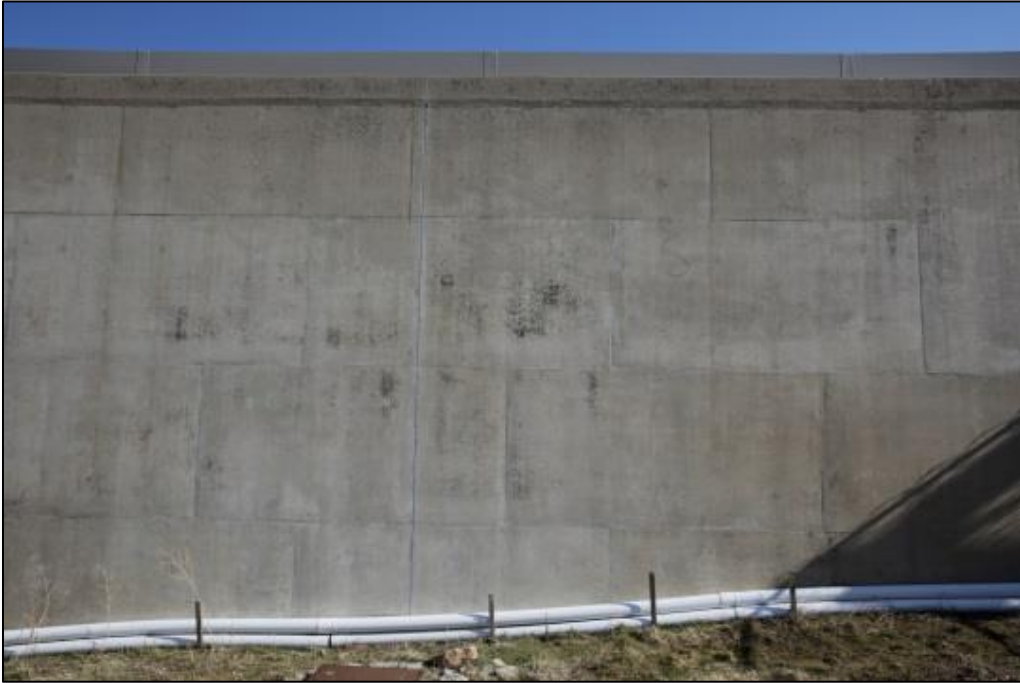
Figure C-2. Exposed Concrete Wall on West Elevation of Auditorium (view southeast)
