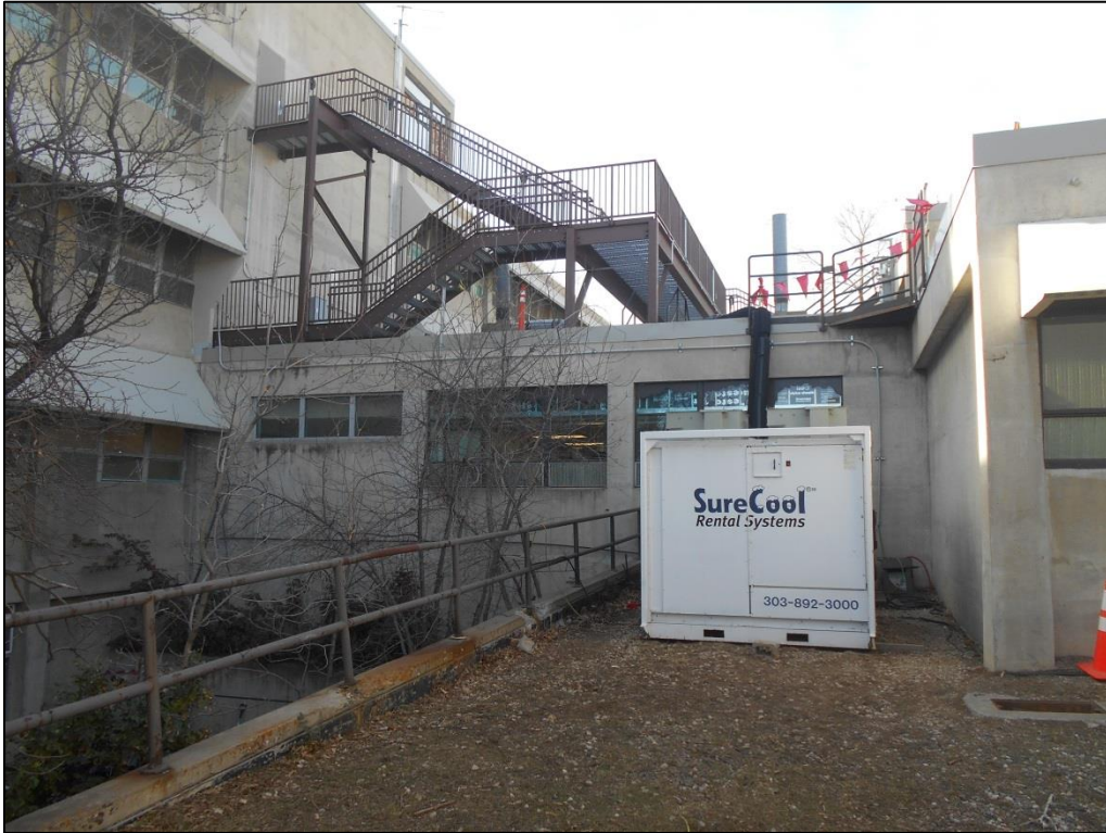
Photo C-32. 2017 Egress Stairway and Secondary Means of Egress on West Side of Penthouse and Spine (view southwest)
