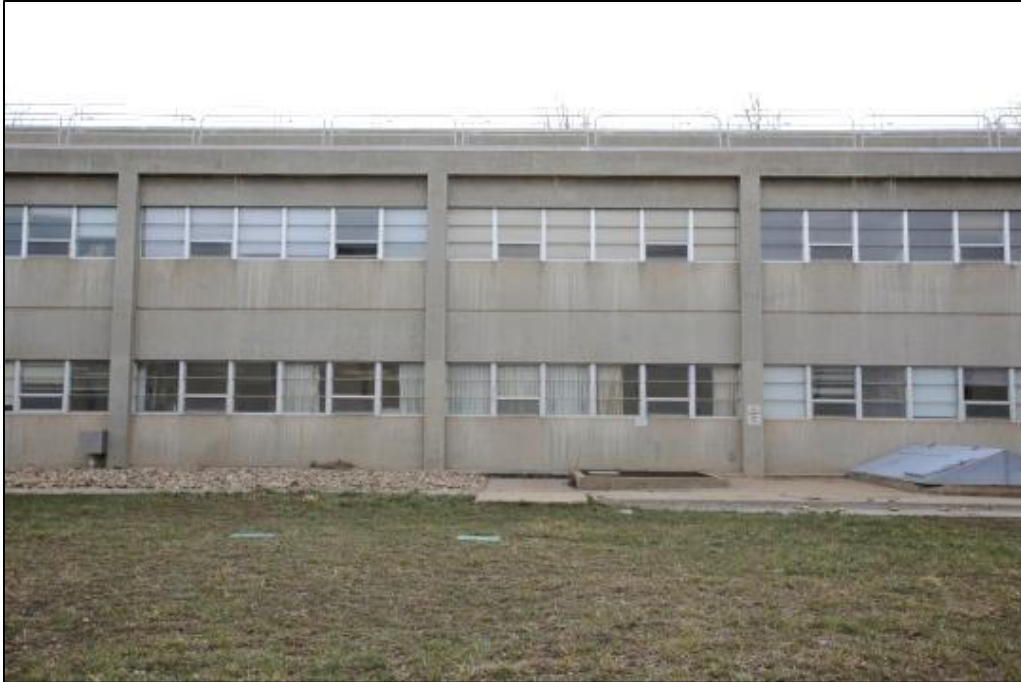
Photo C-65. Wing 5, North Elevation (view southwest)
