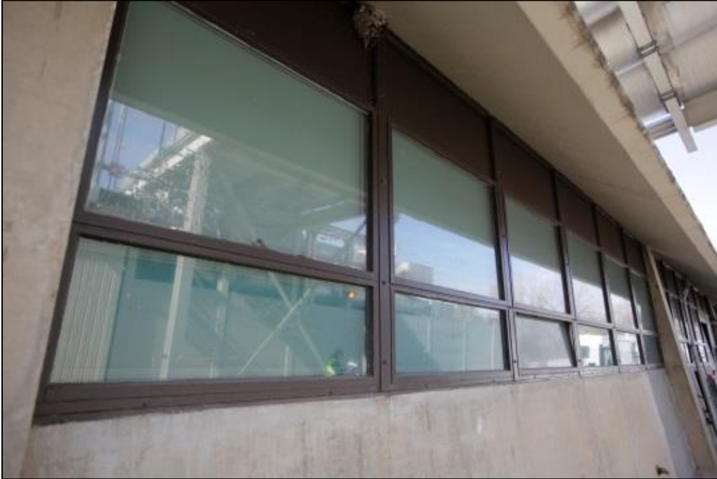
Photo C-38. Original Windows on North Elevation of Wing 1
