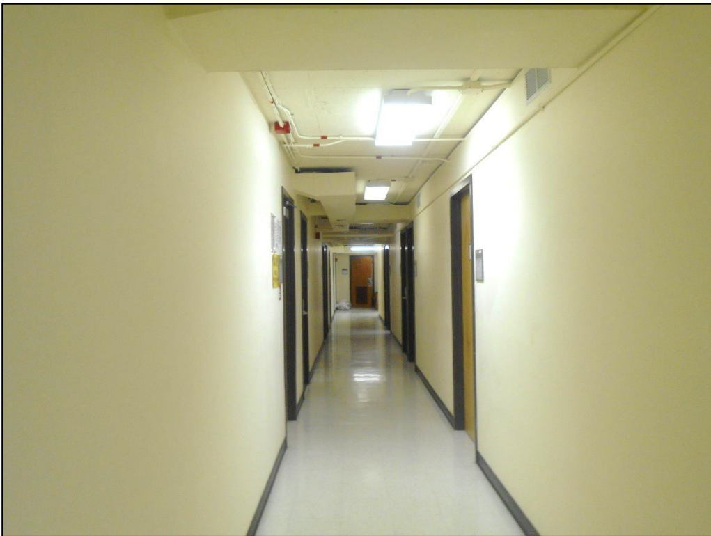
Photo C-148. Basement of Wing 5.
