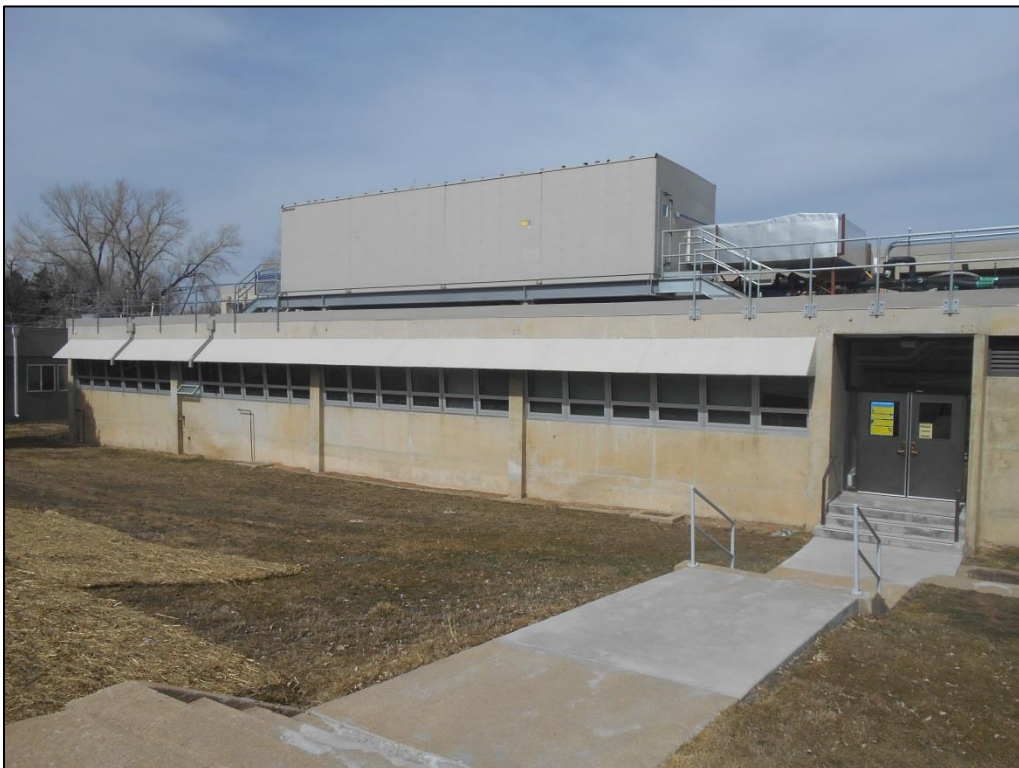
Photo C-36. Replacement Windows and Original Door on South Elevation of Wing 1 (view north)
