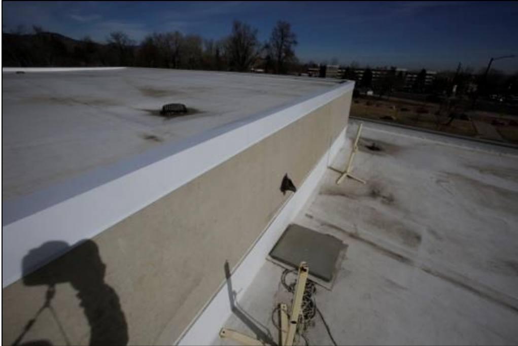
Figure C-13. Roof Drains and Membrane on Auditorium Roof (view northeast)
