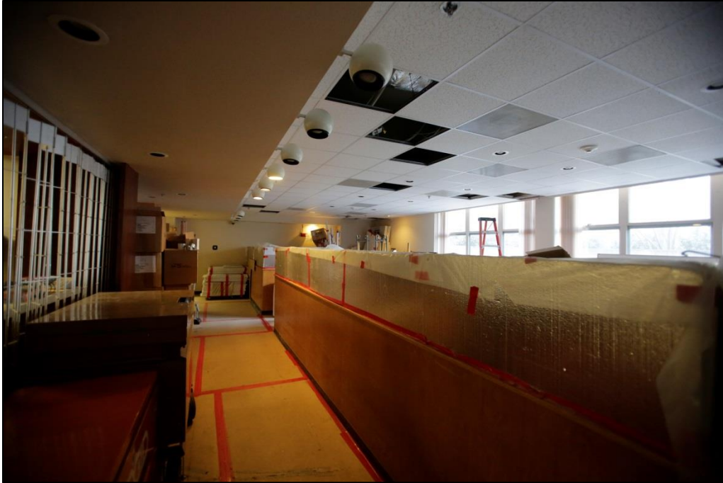
Photo C-119. Former Cafeteria in Level 1 of the Spine (view southwest)
