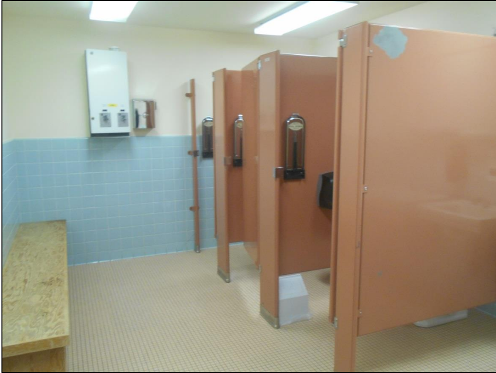
Photo C-149. Women's Restroom in Basement of Wing 5.
