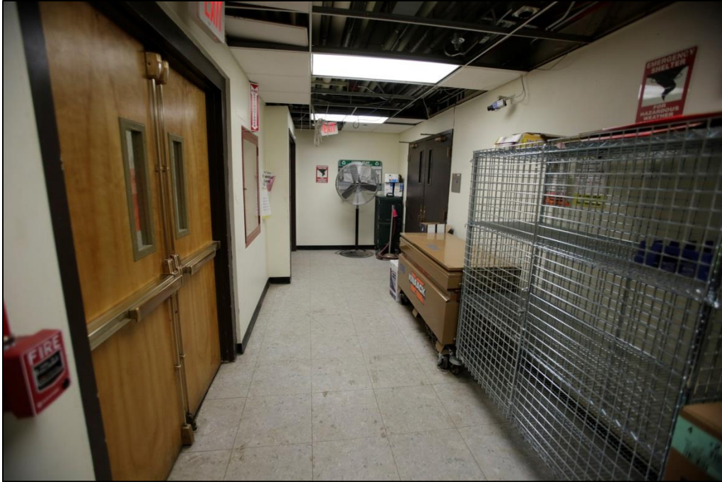
Photo C-121. Corridor between Former Cafeteria Area and Boiler Room (view southwest)
