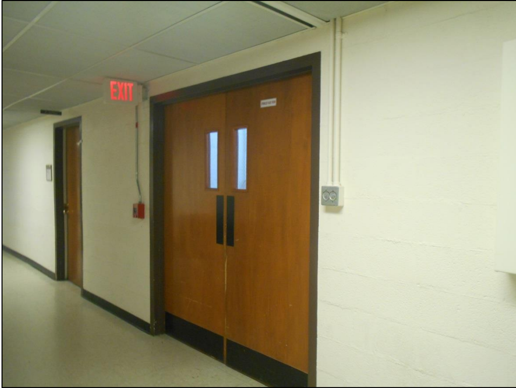
Photo C-143. Original Doors in Wing 2
