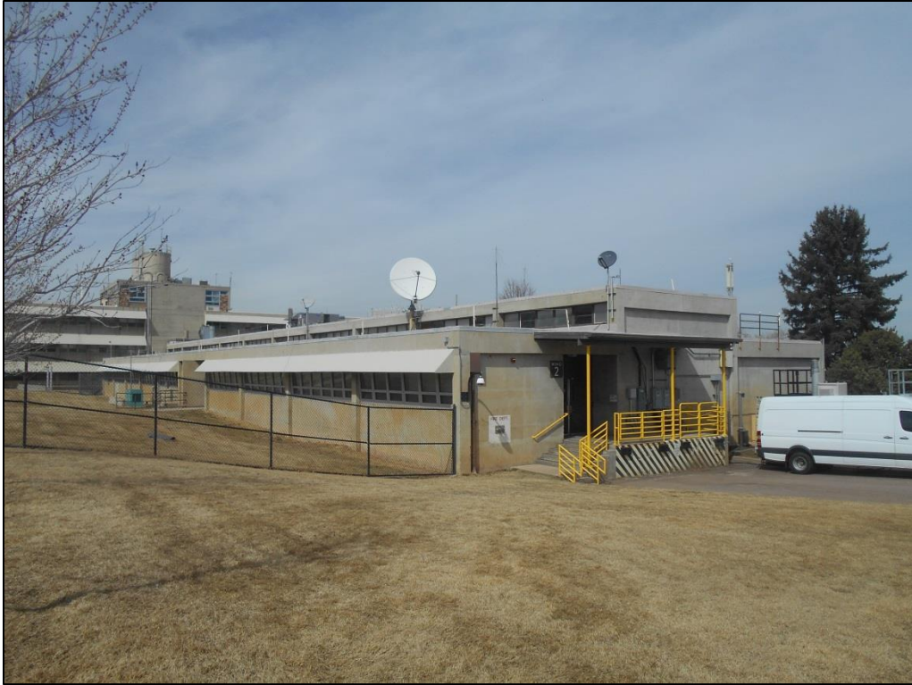
Photo C-47. South and East Elevations of Wing 2 (view north)
