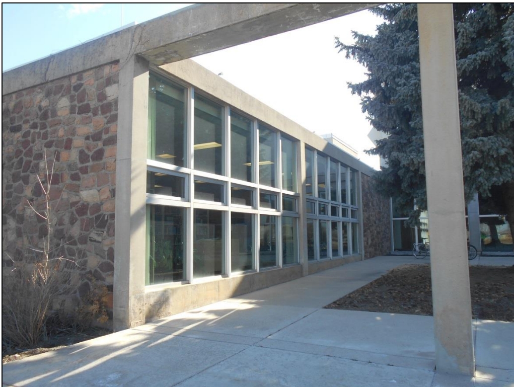
Photo C-16. West Elevation of Library (view south)
