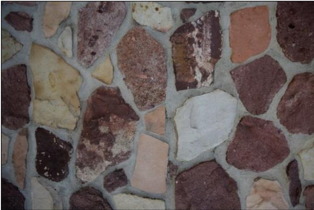
Figure C-4. Detail of Auditorium Stone Wall
