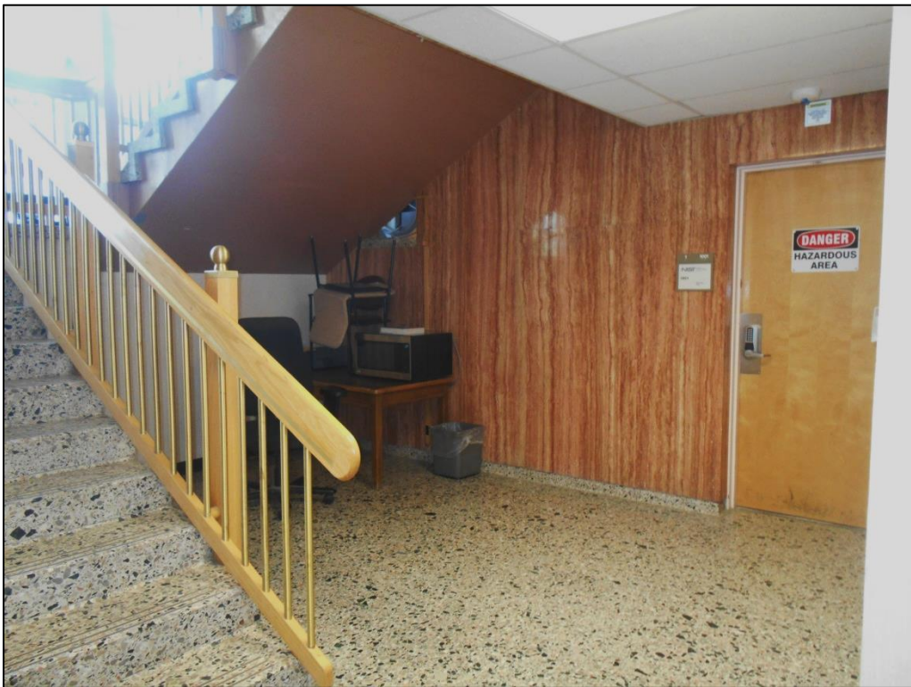
Photo C-106. Lobby Area in Level 1 of the Spine (view southwest)
