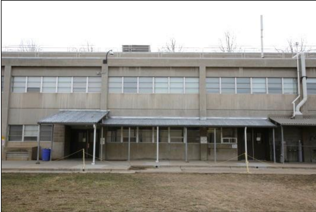
Photo C-67. Metal Awnings on North Elevation (view southwest)
