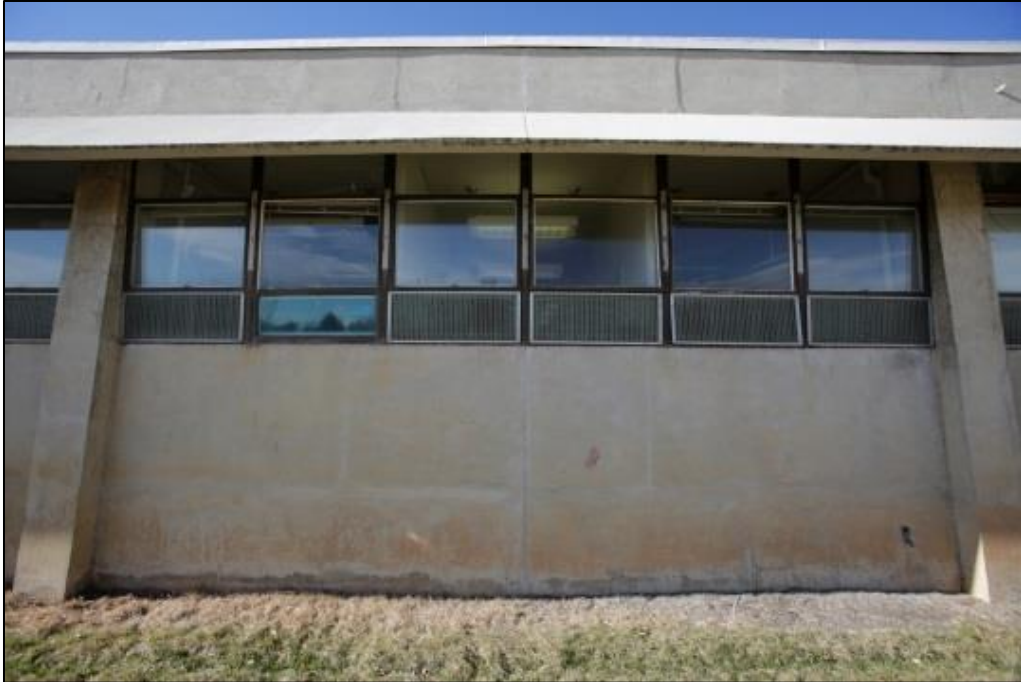
Photo C-59. Typical Wing 4 Exterior Bay (view southwest)
