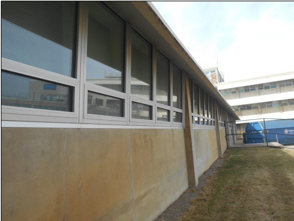
Photo C-50. Replacement Windows on North Elevation of Wing 2 (view northwest)
