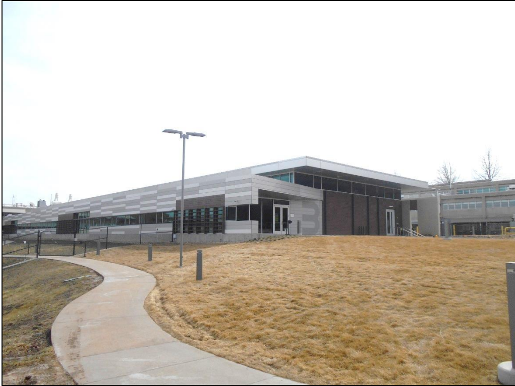
Photo C-57. North and West Elevations of Wing 3 (view south)
