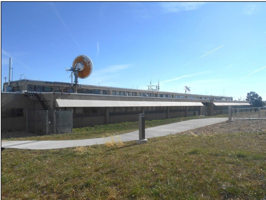
Photo C-60. South Elevation of Wing 4 (view east)
