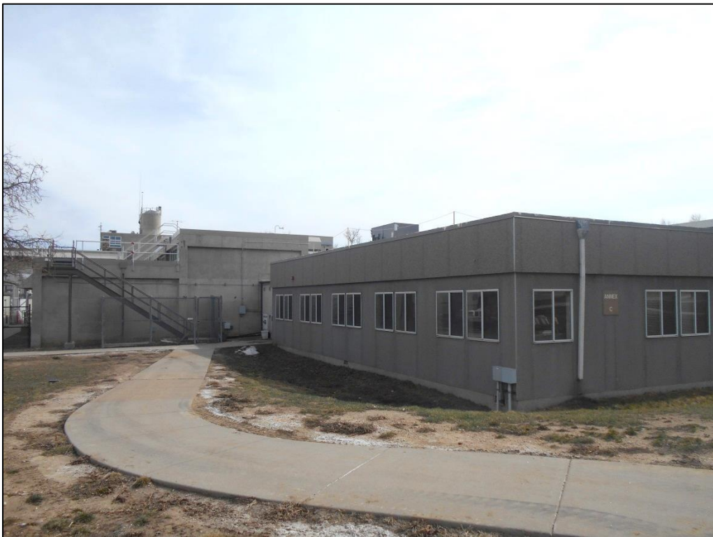
Photo C-42. Annex C and Connecting Hyphen on the West Side of Wing 1 (view southeast)
