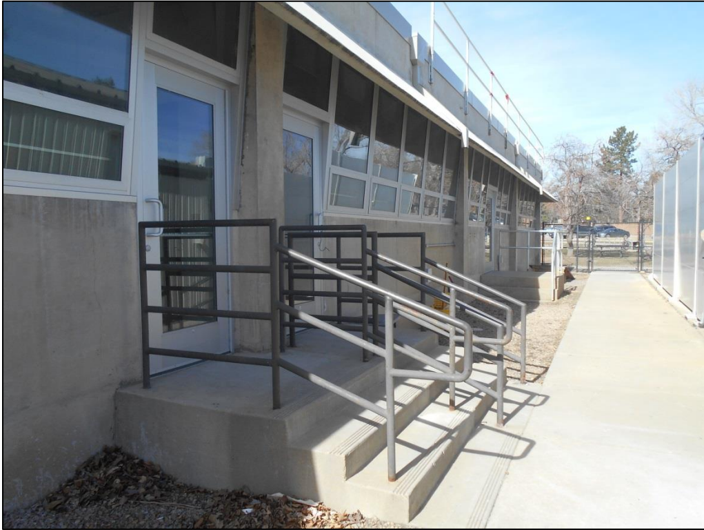
Photo C-40. Replacement Doors on North Elevation of Wing 1 (view southwest)
