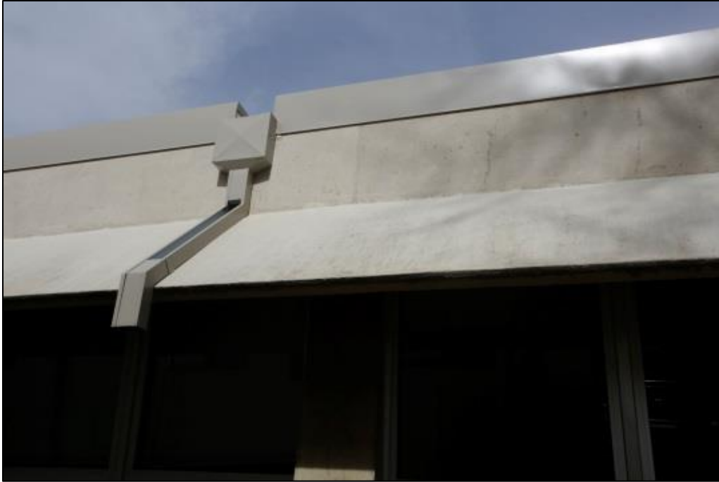
Photo C-41. Downspouts on Wing 1
