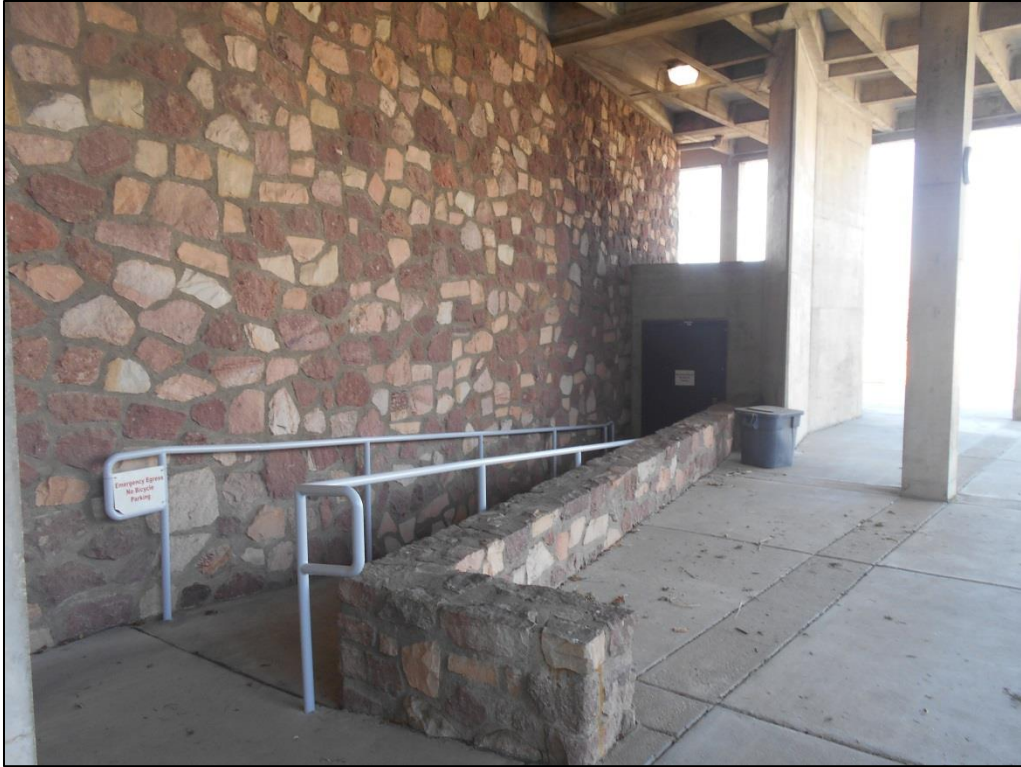
Figure C-9. Ramp to East Auditorium Stage Door, Stone and Brick Retaining Wall, and “Butterfly” Screen Wall (view northeast)
