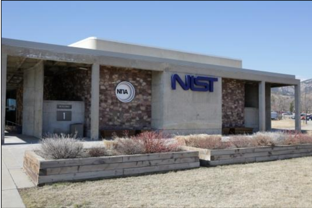
Figure C-7. Concrete Structure and Stone Walls on North Elevation of Auditorium (view southwest)
