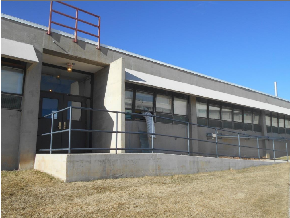
Photo C-62. Door on North Elevation (view west)
