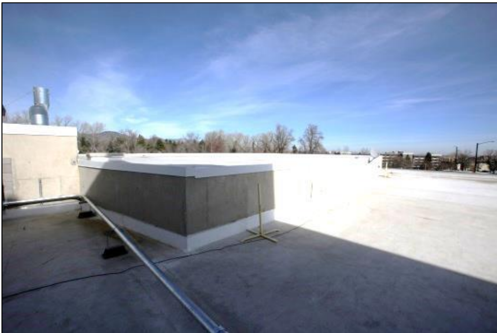
Photo C-12. Roof over Auditorium (view northeast)
