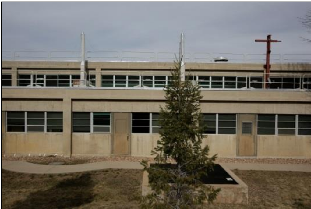
Photo C-66. Wing 5, South Elevation (view northeast)
