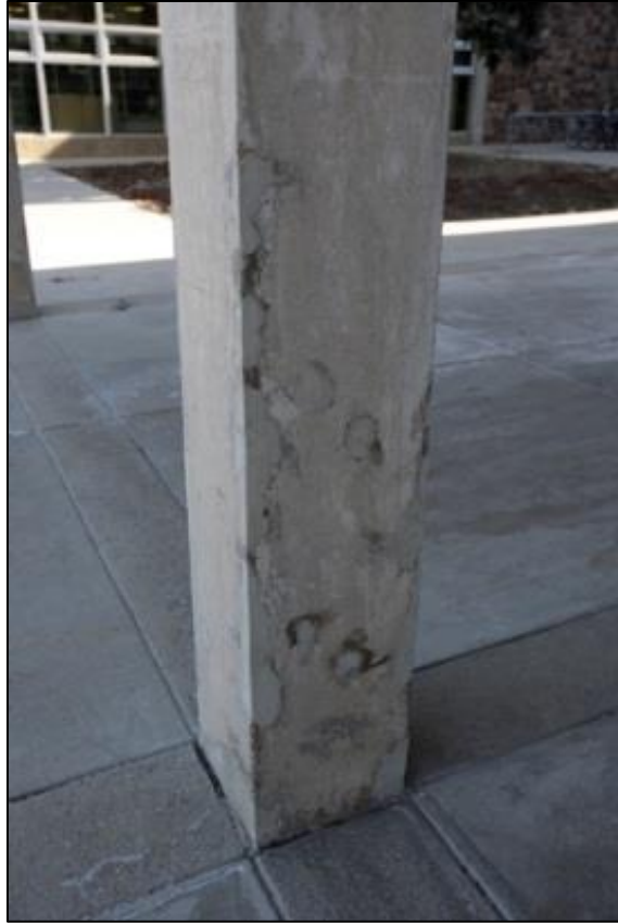
Photo C-23. Patched Columns in Courtyard
