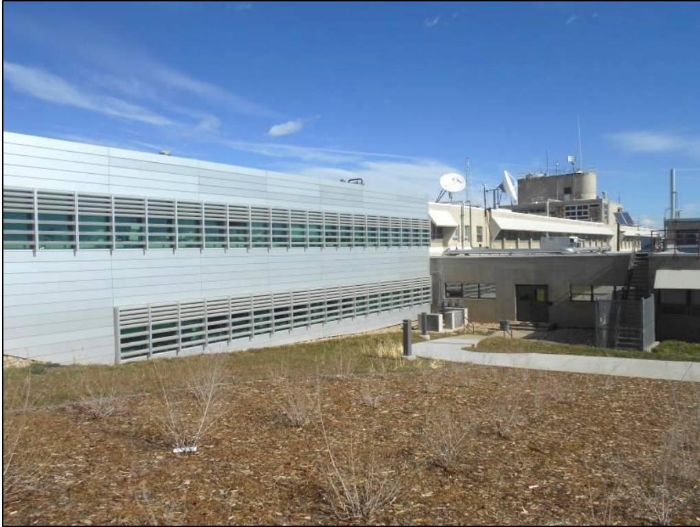
Photo C-33. South Elevation of the Spine between Wings 4 and 6 (view north)
