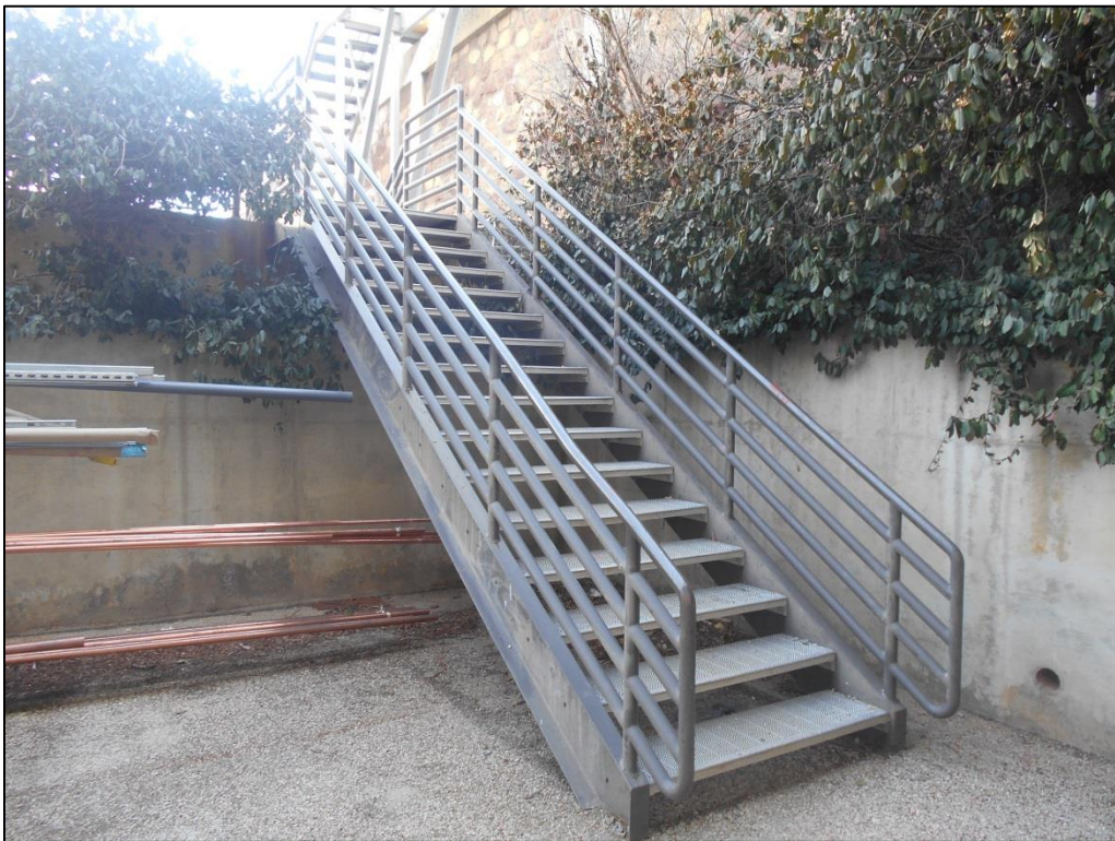
Photo C-120. Modern Metal Staircase in Sunken Terrace (view north)
