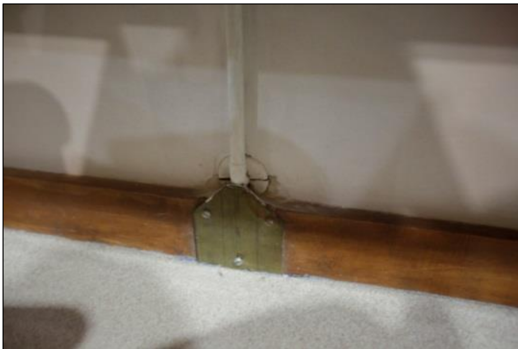
Photo C-76. Detail of Base on East and West Walls
