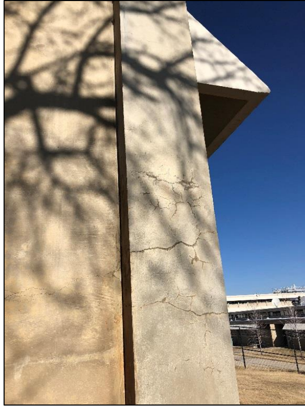
Photo C-163. Column Cracks
