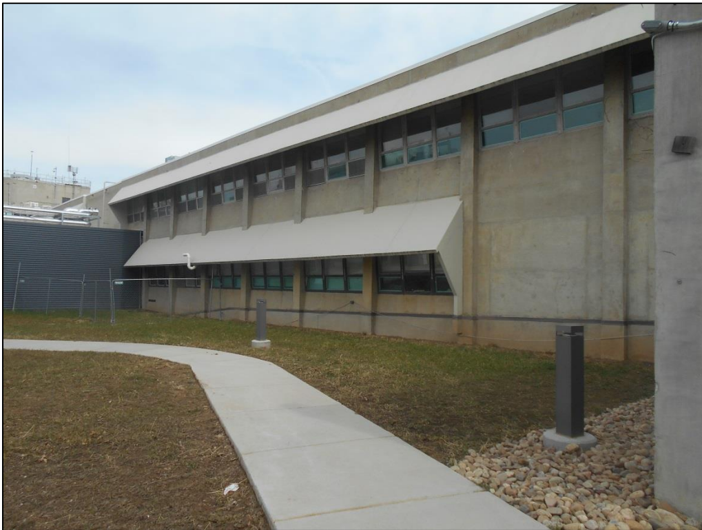
Photo C-26. West Elevation of Spine between Wings 3 and 5 (view northeast)
