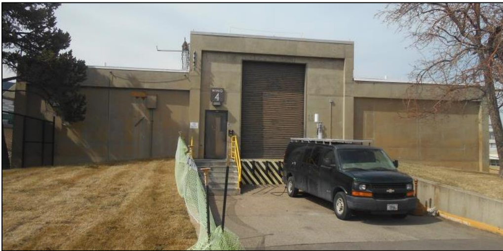
Photo C-64. Wing 4, South Elevation (view northwest)
