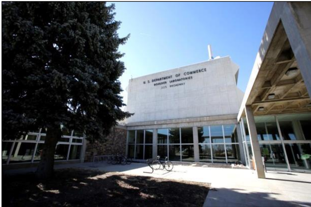
Photo C-20. Building 1 Courtyard and Main Entrance to Lobby (view southwest)
