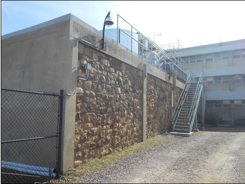
Figure C-11. South Wall of Auditorium (view east)
