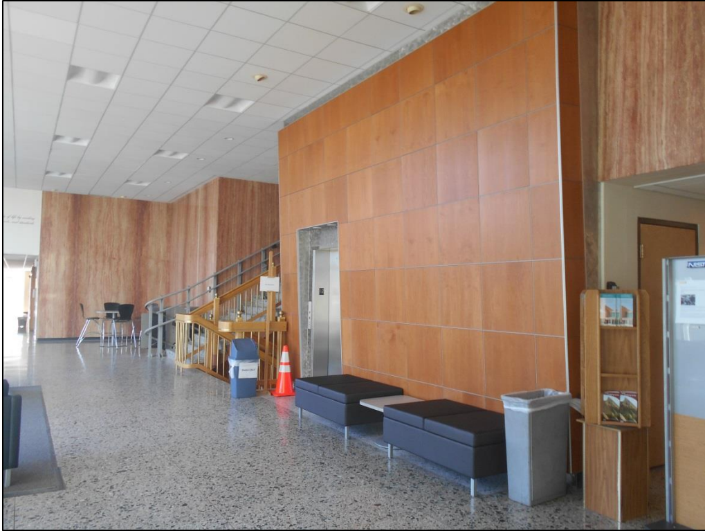
Photo C-97. South Wall of Lobby (view southeast)
