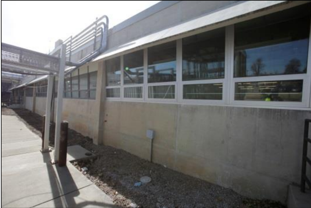
Photo C-35. Original and Replacement Windows on North Elevation of Wing 1 (view southeast)
