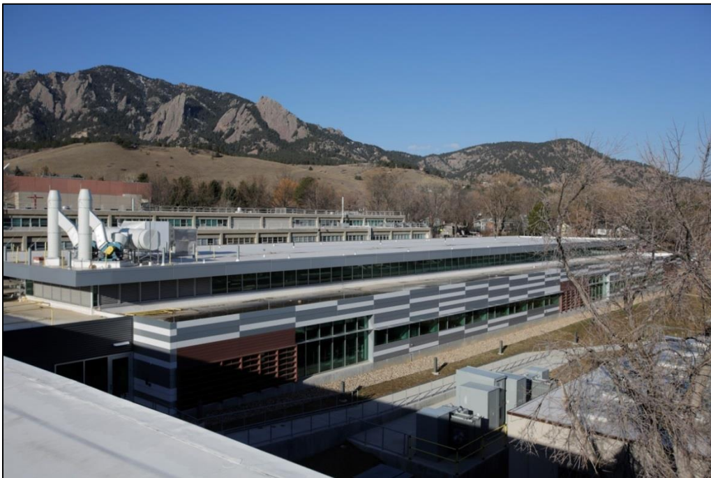
Photo C-56. North Elevation of Wing 3 (view west).
