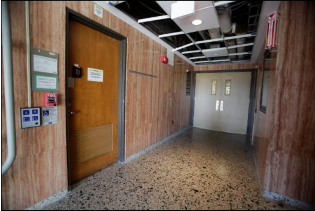
Photo C-105. Lobby Area in Level 2 of the Spine (view southwest)
