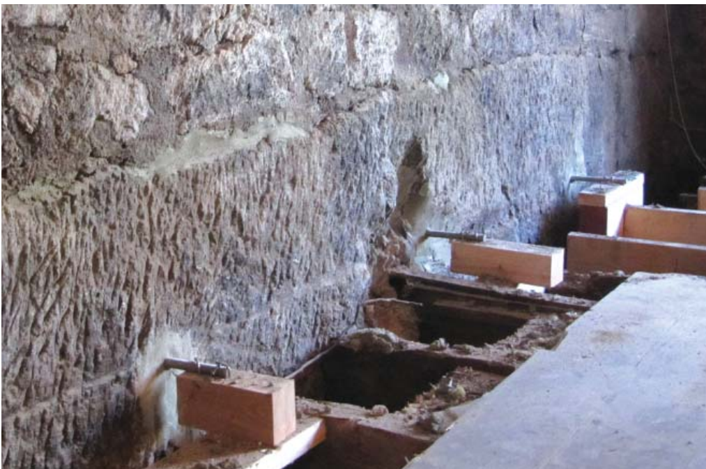
Figure 24. Eye bolts used to anchor the floor to the wall.
