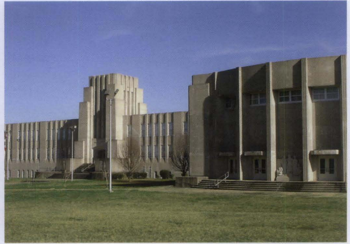
Figure 6. The Bailey Magnet School in Jackson, Mississippi, was designed as the Jackson Junior High School by the firm of N.W. Overstreet & Town in 1936. The streamlined building exemplifies the applicability of concrete to creating a modern architectural aesthetic. Photo: Bill Burris, Burris/Wagnon Architects, P.A.
