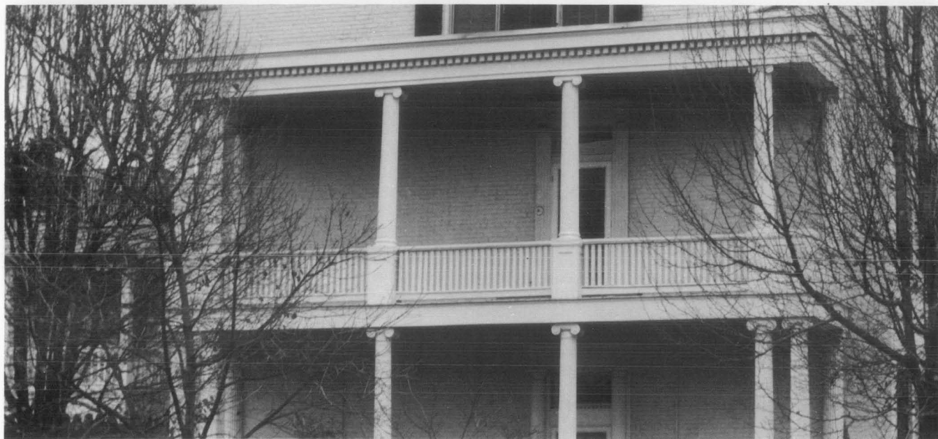
Columns were repaired and a capital was replaced in epoxy on this 19th-century 2-story porch. Photo: Dell Corporation
