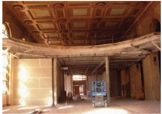
Figure 12. A mezzanine was added to the original banking hall of this 1921 former bank building as a seismic strengthening measure. Subdividing such an important character-defining space can result in a severe loss to a building's historic integrity.
