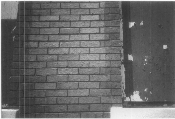
Figure 18. The glazed bricks in the center of the pier were covered by a signboard that protected them from being damaged by the sandblasting which removed the glaze from the surrounding bricks.
