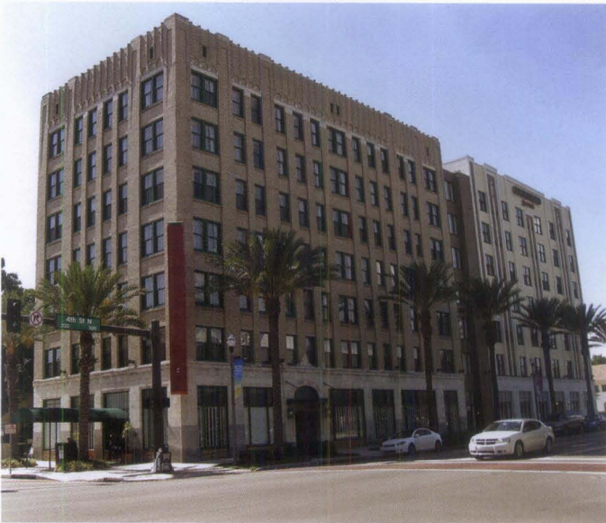
Figure 2. The new section on the right is appropriately scaled and reflects the design of the historic Art Deco-style hotel. The apparent separation created by the recessed connector also enables the addition to be viewed as an individual building.
