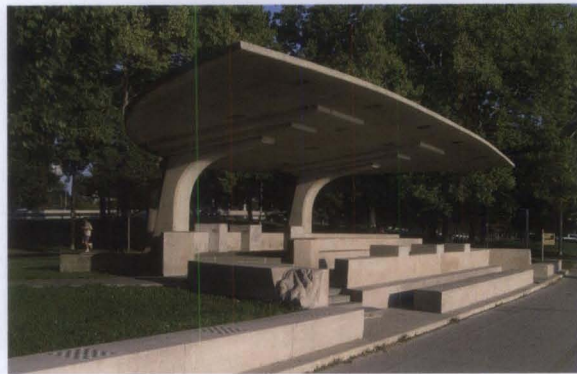
Figure 8. The Chess Pavilion in Chicago's Lincoln Park was designed by architect Morris Webster and constructed in 1956. The pavilion is a distinctive landscape feature, with its reinforced concrete cantilevered slab that provides cover for chess players.
