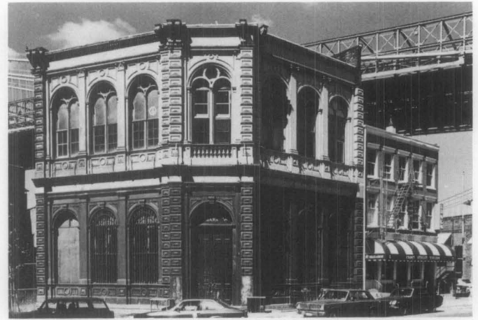
Illus. 4. The 19th-century also produced a variety of metal products used in imitation of other materials. In this case, the entire exterior of the Long Island Safety Deposit Company is cast-iron representing stone. Photo: Becket Logan, Friends of Cast Iron Architecture.
