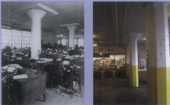
Figure 11. Whether in a circa 1925 office (left) or in a parking garage and retail facility (right), exposed concrete structures help characterize these building interiors. Photo: Minnesota Historical Society (left).
