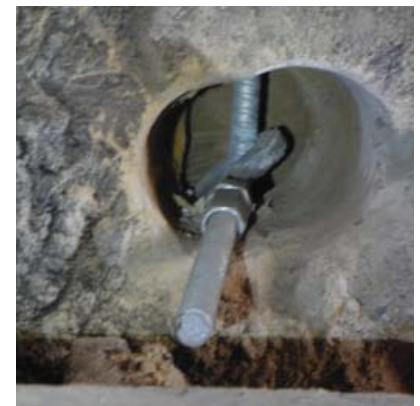
Figure 24. Eye bolts used to anchor the floor to the wall.
