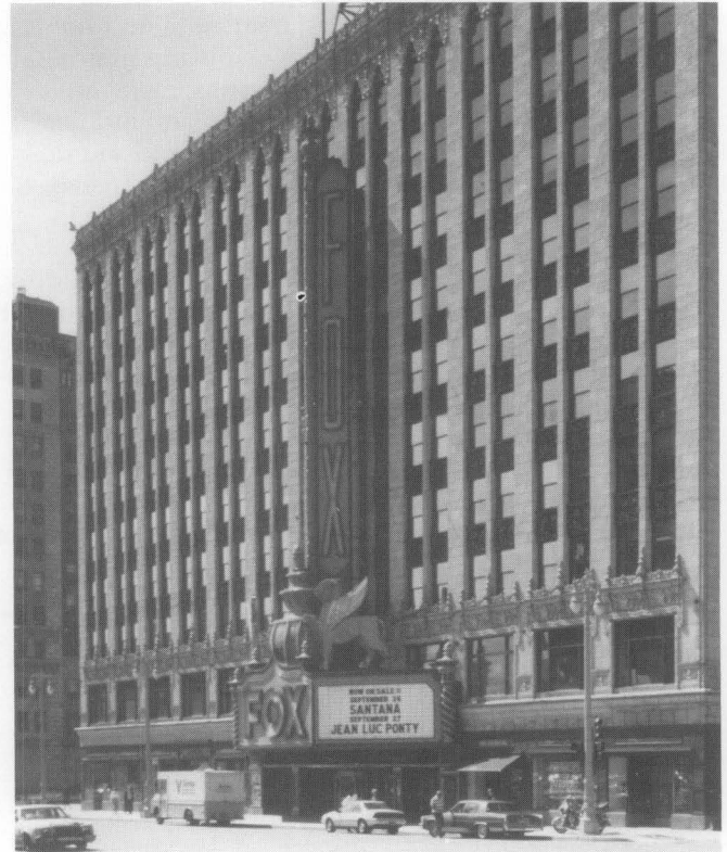
3. The circa 1928 Fox Theater in Detroit, designed by C. Howard Crane, was one of the earliest twentieth century buildings to provide air conditioning to its patrons. The early water-cooled system was recently restored. Commercial and highrise buildings of the twentieth century were able, mostly through electrical power, to provide sophisticated systems that integrated many building services. Photo: William Kessler and Associates, Architects.
