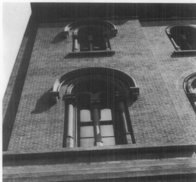
Illus. 8. Even when materials are not locally available, it may be possible and cost effective to find sources elsewhere. For example, the local sandstone was no longer available for the restoration of the New York Shakespeare Festival Public Theater. The deteriorated sandstone window hoods, were replaced with stone from Germany that closely matched the color and texture of the historic sandstone. Photo: John G. Waite.
