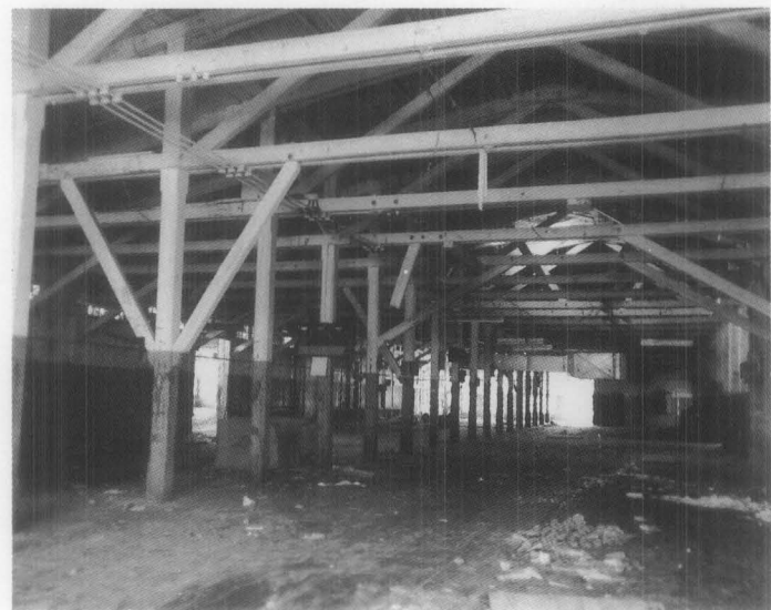
Figure 2. The interiors of mills and industrial buildings frequently are open, unadorned spaces with exposed structural elements. While the new uses to which this space could be put are many—retail, residential, or office—the generous floor-to-ceiling height and exposed truss system are important character-defining features and should be retained in the process of rehabilitation.
