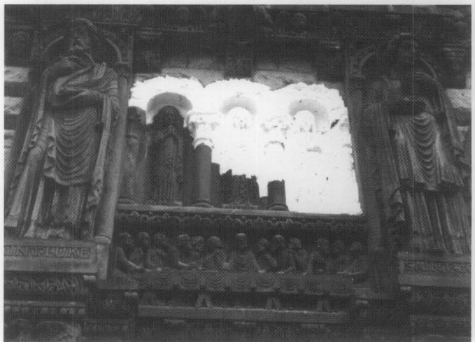
Figure 17. A poultice is being used to remove salts from the brownstone statuary on the facade of this late-19th century stone church. Photo: National Park Service Files.
