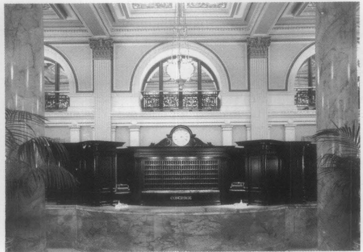
Figure 11. These dramatic "before" and "after" photographs show a severely deteriorated space restored to its original elegance: plaster has been repaired and painted, the scagliola columns have been restored to match marble using traditional craft techniques, and missing decorative metalwork has been re-installed in front of the windows. Although some reorganization of the space took place, notably the relocation of the front desk, the overall historic character of the space has been preserved. These views are of the lobby in the Willard Hotel, Washington, D.C. Credit: Commercial Photographers (left); Carol M. Highsmith (right)
