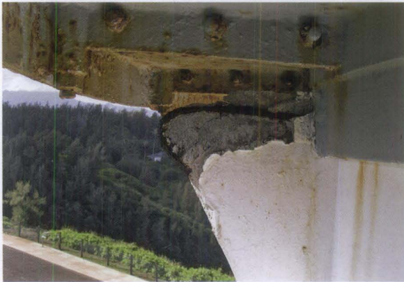
Figure 12. The concrete lighthouse at the Kilauea Point Light Station, Kilauea, Kauai, Hawaii, was constructed circa 1913. The concrete, which was a good quality, high strength mix for its day, is in good condition after almost one hundred years in service. Deterioration in the form of spalling related to corrosion of embedded reinforcing steel has occurred primarily in areas of higher ornamentation such as projecting bands and brackets (see close-up photo).
