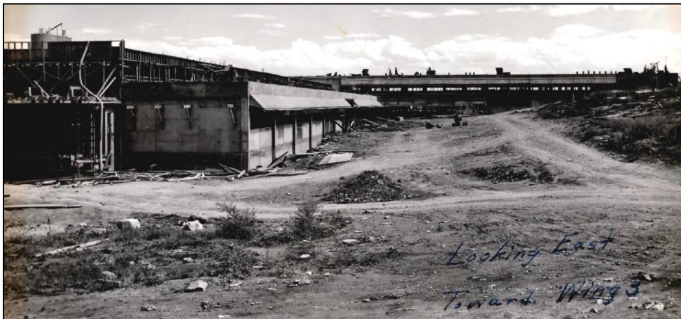
Figure 2-5. Wing 3 and Spine under Construction, September 1, 1953, view southeast (photograph courtesy of Department of Commerce Boulder Laboratories)
