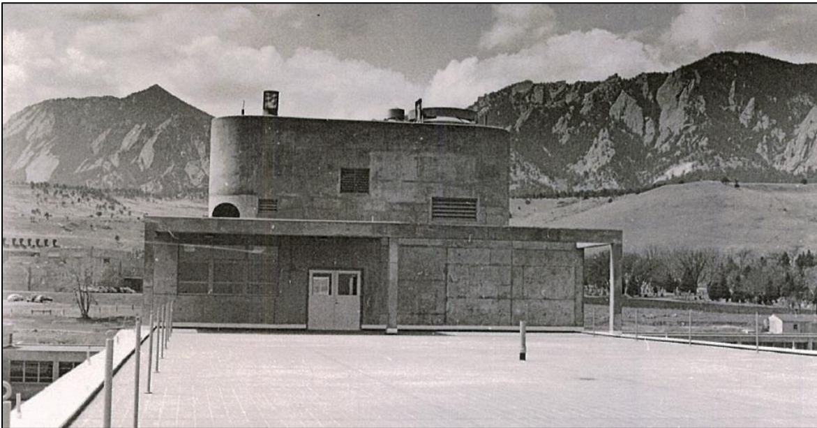
Figure 2-15 Rooftop Penthouse and Boiler Stack, 1954 (view southwest; photograph courtesy of Carnegie Library for Local History, Boulder, Colorado, Museum of Boulder Collection)
