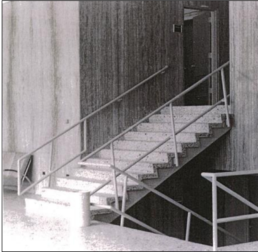
Figure 2-38. Staircases to Levels 1 and 2 of the Spine in May 1954 looking southeast toward the Library (photograph courtesy of Carnegie Library for Local History, Boulder, Colorado, Museum of Boulder Collection)
