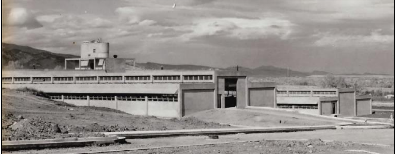
Figure 2-31. South and East Elevations of Wings 4 and 2, November 2, 1953 (view northwest; cropped to show detail; photograph courtesy of Department of Commerce Boulder Laboratories)
