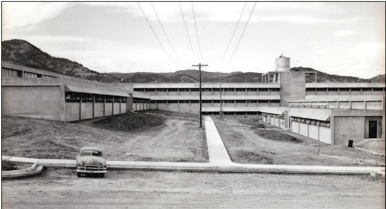
Figure 2-30. North Elevation of Wing 4, East Elevation of the Spine, and South Elevation of Wing 2, November 1953 (view northwest; photograph courtesy of Department of Commerce Boulder Laboratories)
