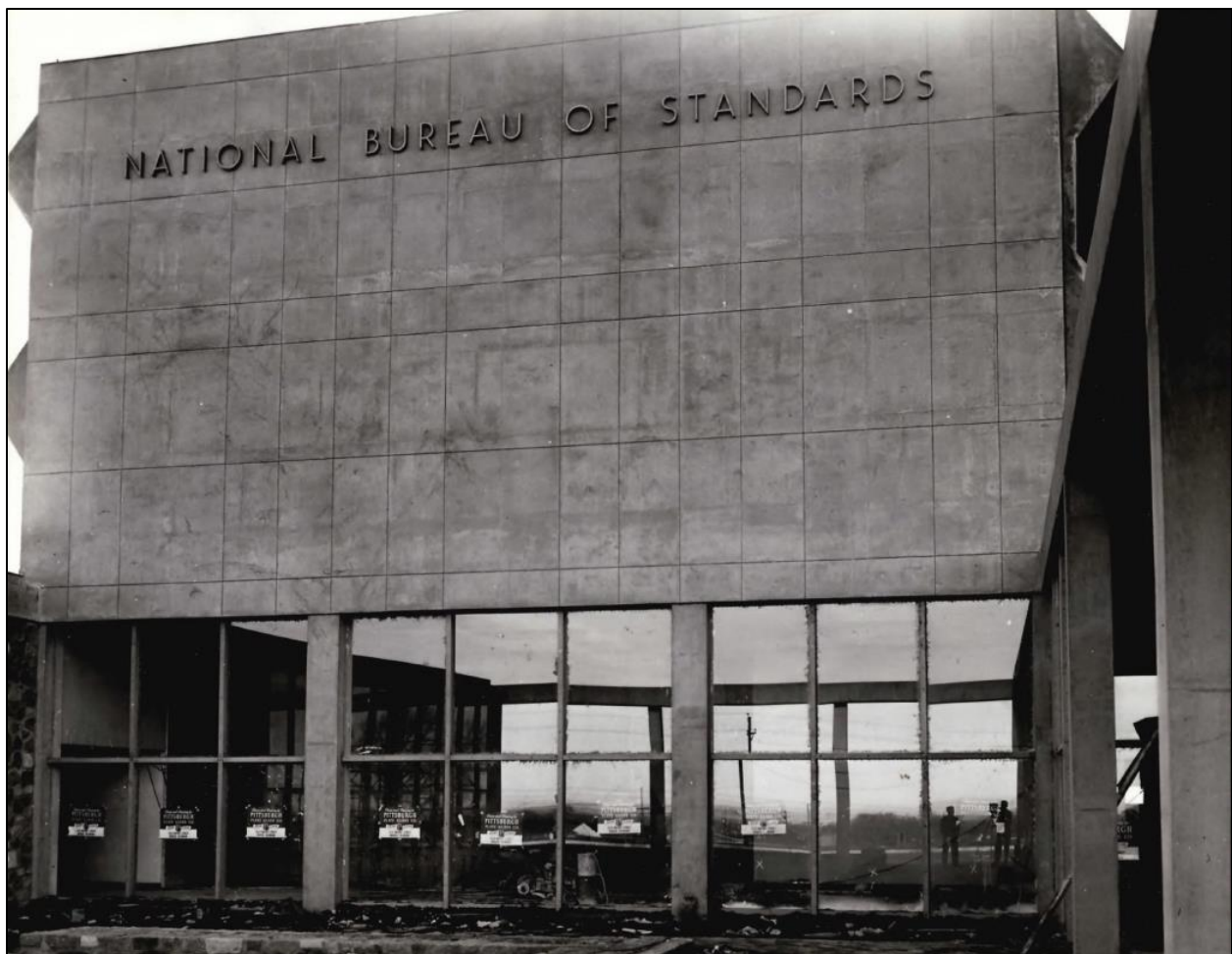
Figure 2-19. North End of the Spine at the Front of the House, January 31, 1954 (view southwest; photograph courtesy of Department of Commerce Boulder Laboratories)
