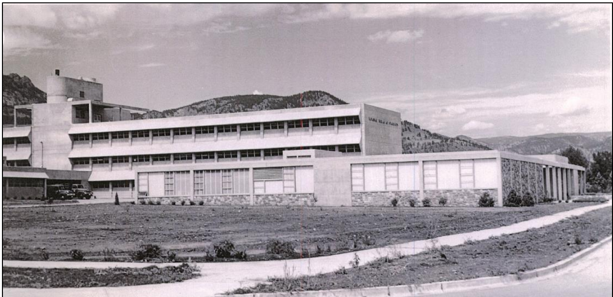
Figure 2-21. East Elevation of the Library at the Front of the House in 1954 (view west; photograph courtesy of Carnegie Library for Local History, Boulder, Colorado, Museum of Boulder Collection)
