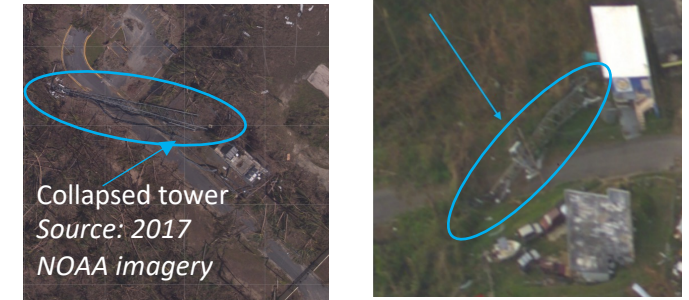
Wireless comm: cell tower collapse
