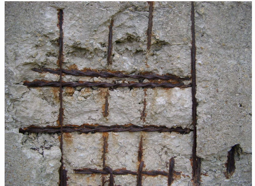
Rebar in concrete
