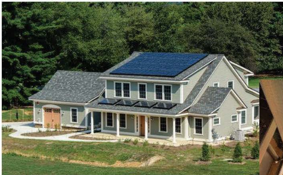
Net-zero Energy Research Facility
