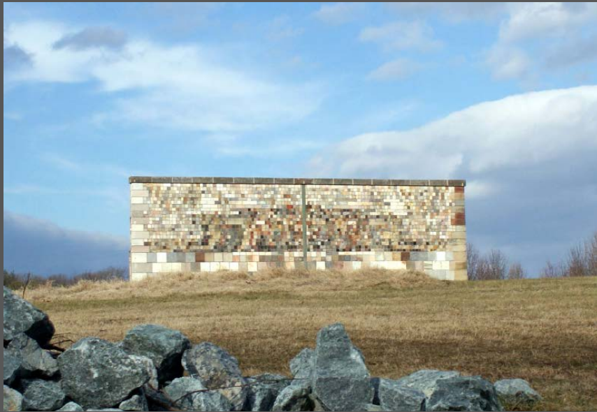
Masonry Test Wall
