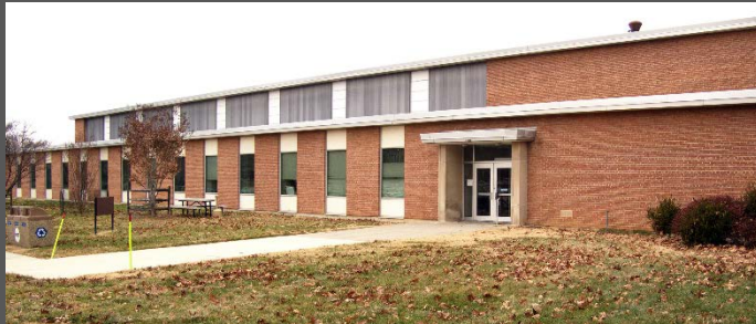
Building 304: Shops (Instrument)
