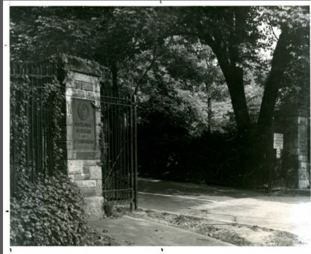
Stone Gate Post and Gate at Upton Street
