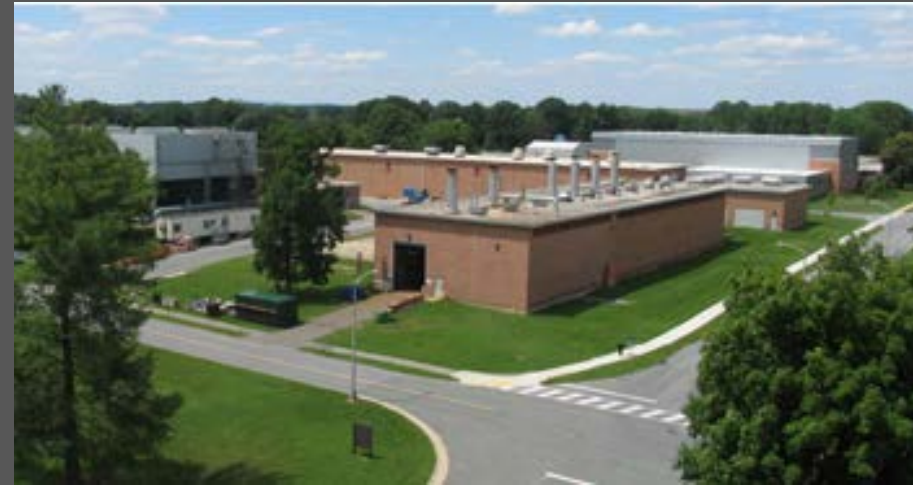
Building 302: Steam and Chilled Water Plant
