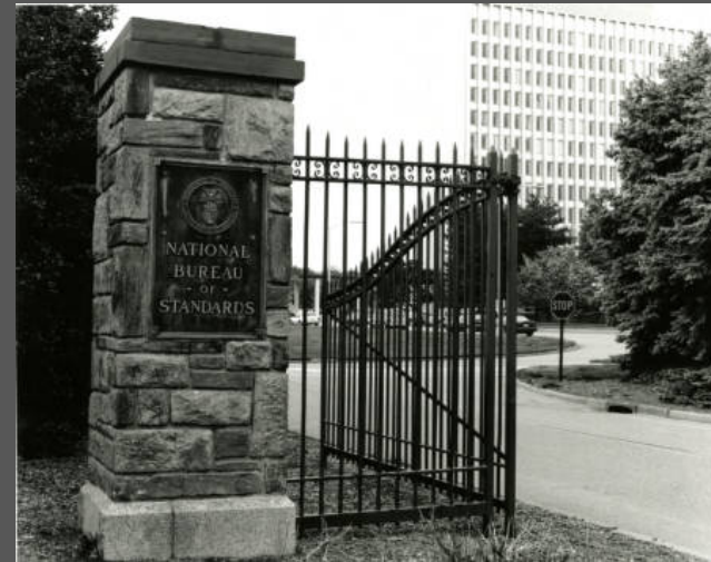
Relocated Post and Gate at Gaithersburg
