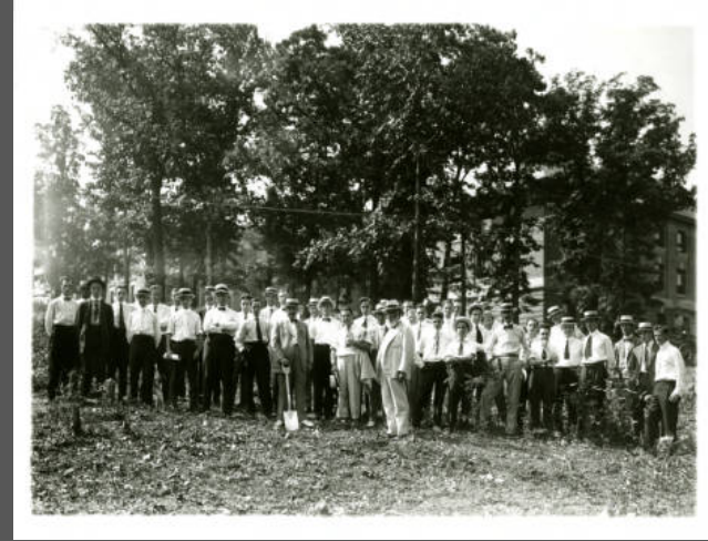
Chemistry Building Ground Breaking, 1916
