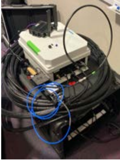
(a) Sensor staged for deployment
