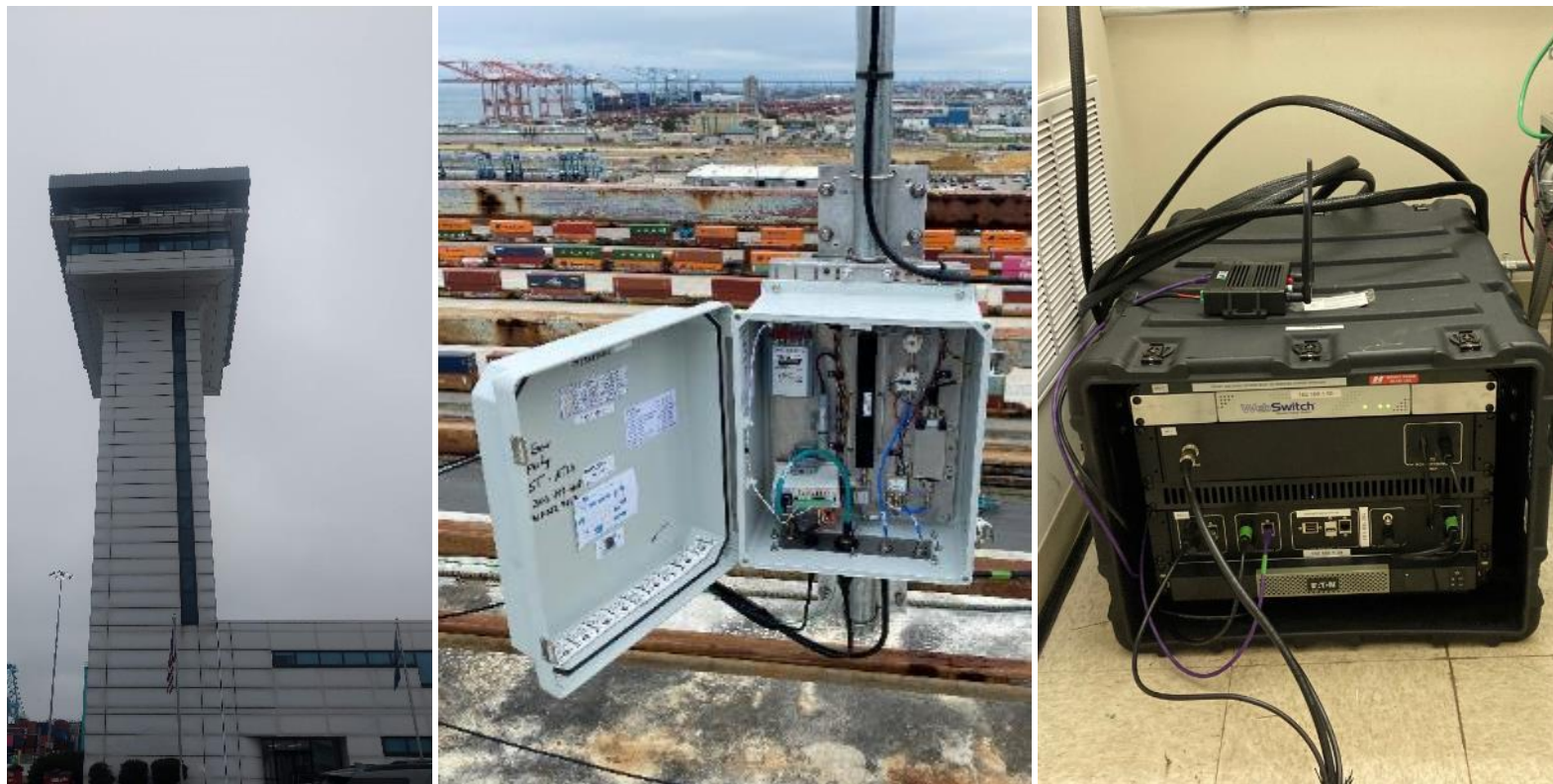
South Tower, Site
