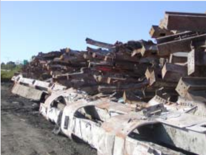
WTC steel columns
