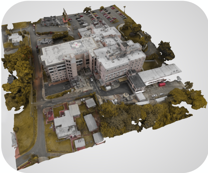
Hospital Bella Vista Point Cloud Model
