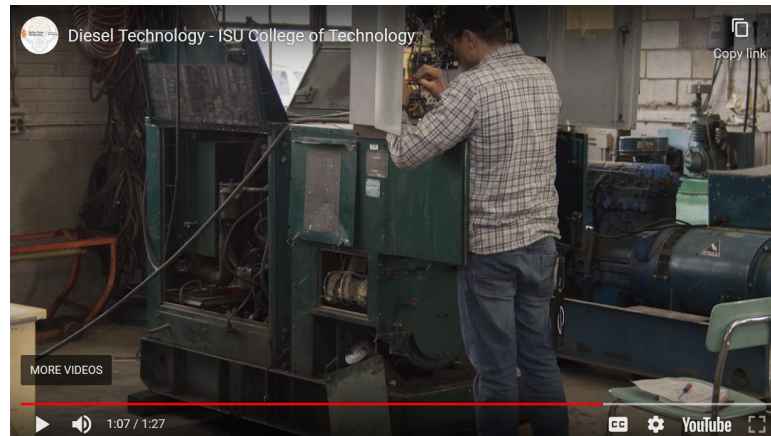
Diesel Power Systems
