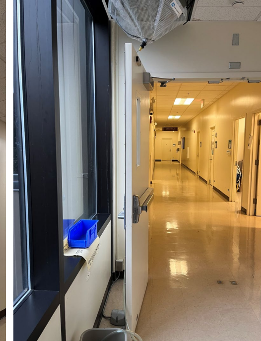
Unresolved water leaks: Leak diverters used as long-term water leak control measures (note that Guide Hall leak diverter is near electrical equipment).
