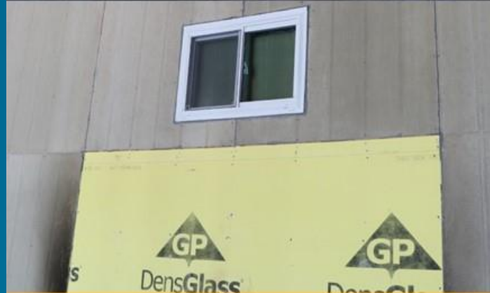
No thermal damage to sheathing
