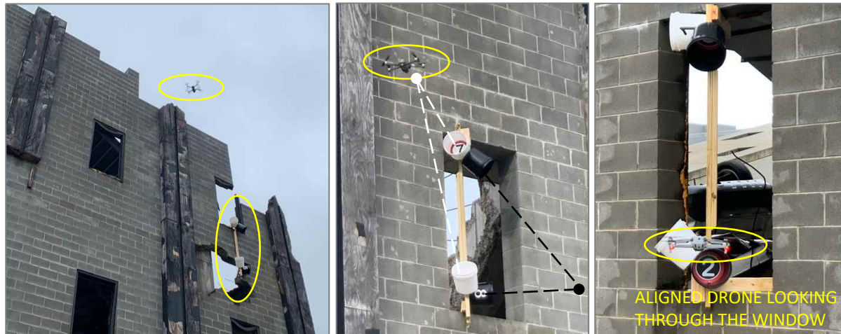
Figure 27) The scenario façade was embedded with window inspection tasks on two sides with partially collapsed walls. Each Dual Bucket Alignment guides the remote pilot to positions and orientations with high/low and left/right views inside the windows.
