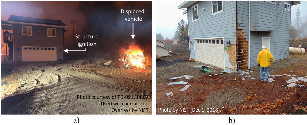
Figure 52. A defended structure on Lewis Ranch Rd where the burning vehicle was igniting the structure, showing a) a dozer displaced the vehicle to stop fire spread, b) the associated evidence of the fire ignition and defensive actions encountered during NIST damage assessments.
