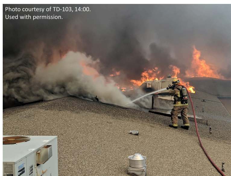
Figure 31. The cardiology section of FRH was destroyed. Extensive firefighting efforts prevented spread to other portions of the facility.
