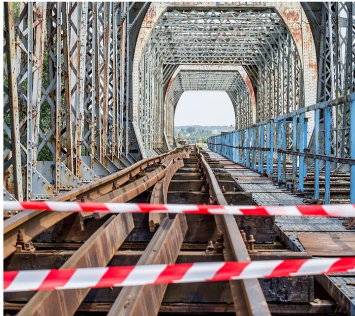
Physical Infrastructure (new)
