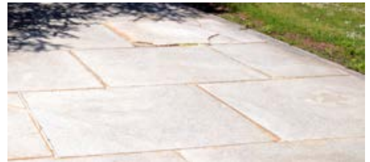
Large white granite pavers—Historic Core
