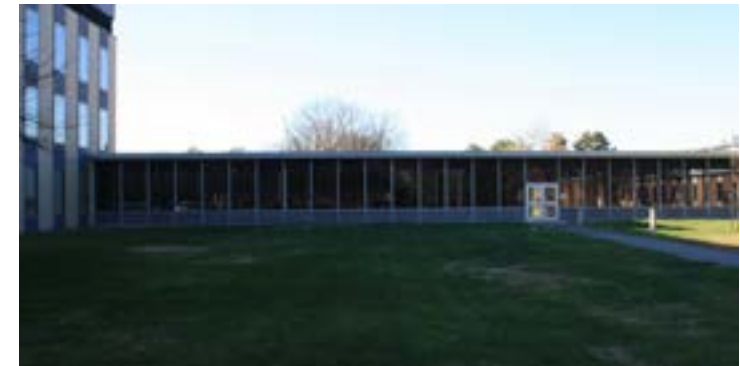
The main internal corridor with a connection to exterior circulation
