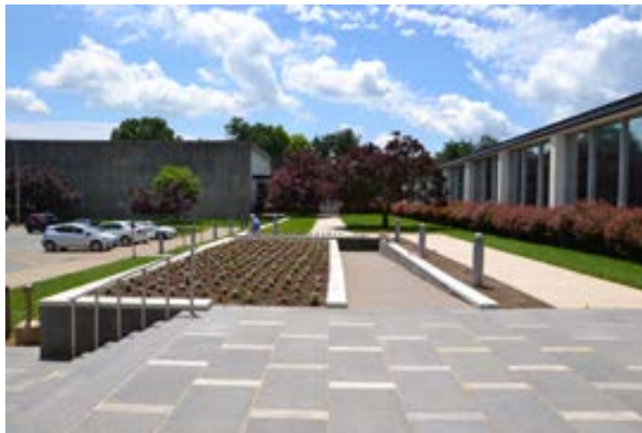
The formal entrance to Building 101.
