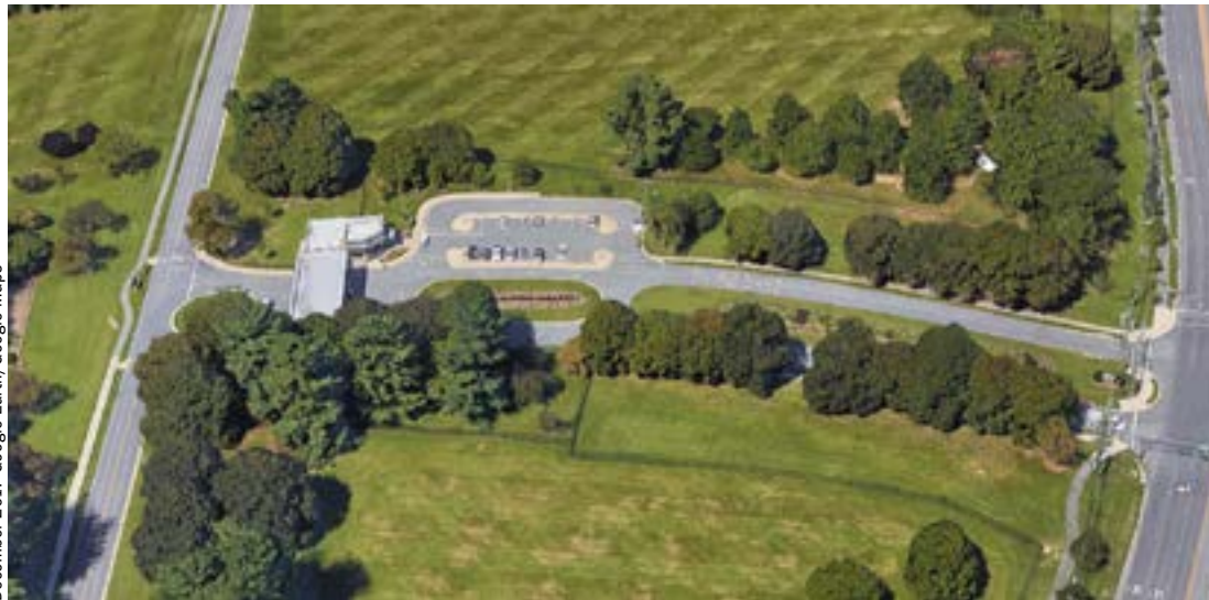
Exhibit 56: Existing Gate A Conditions
