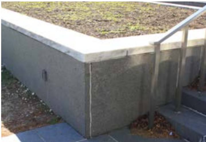
Granite veneer, marble coping, steel handrail—Historic Core
