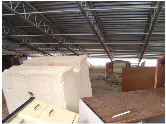
Figure 4. The House of Pancakes viewed from inside.
