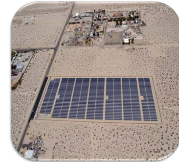
Borrego Springs Utility Grid Reliability Improvements, Respond to Customer Outages Faster, Integration of Renewables
