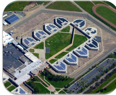
Santa Rita jail Energy Resilience, Cost Savings, GHG Reductions
