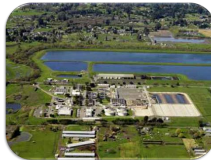
Municipal Facility Increase Reliability, Compete in Grid Markets Lower costs
