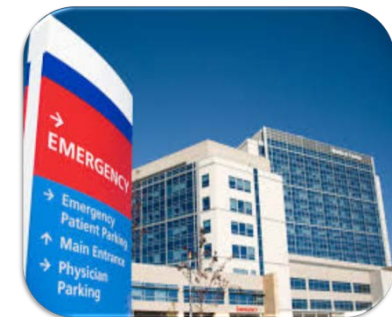
Medical Hospital Increase Reliability, More Flexibility Lower costs
