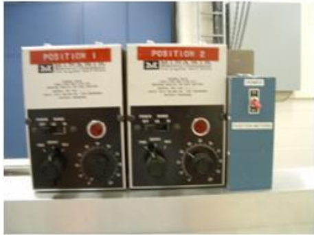
Chamber alignment controls 300 kV range
