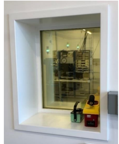
Calibrator status lights visible through the lead glass window
