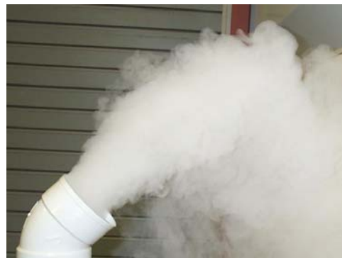
Figure 6: A dense gas-like ultra fine water mist NanoMist® dispersion in a room
