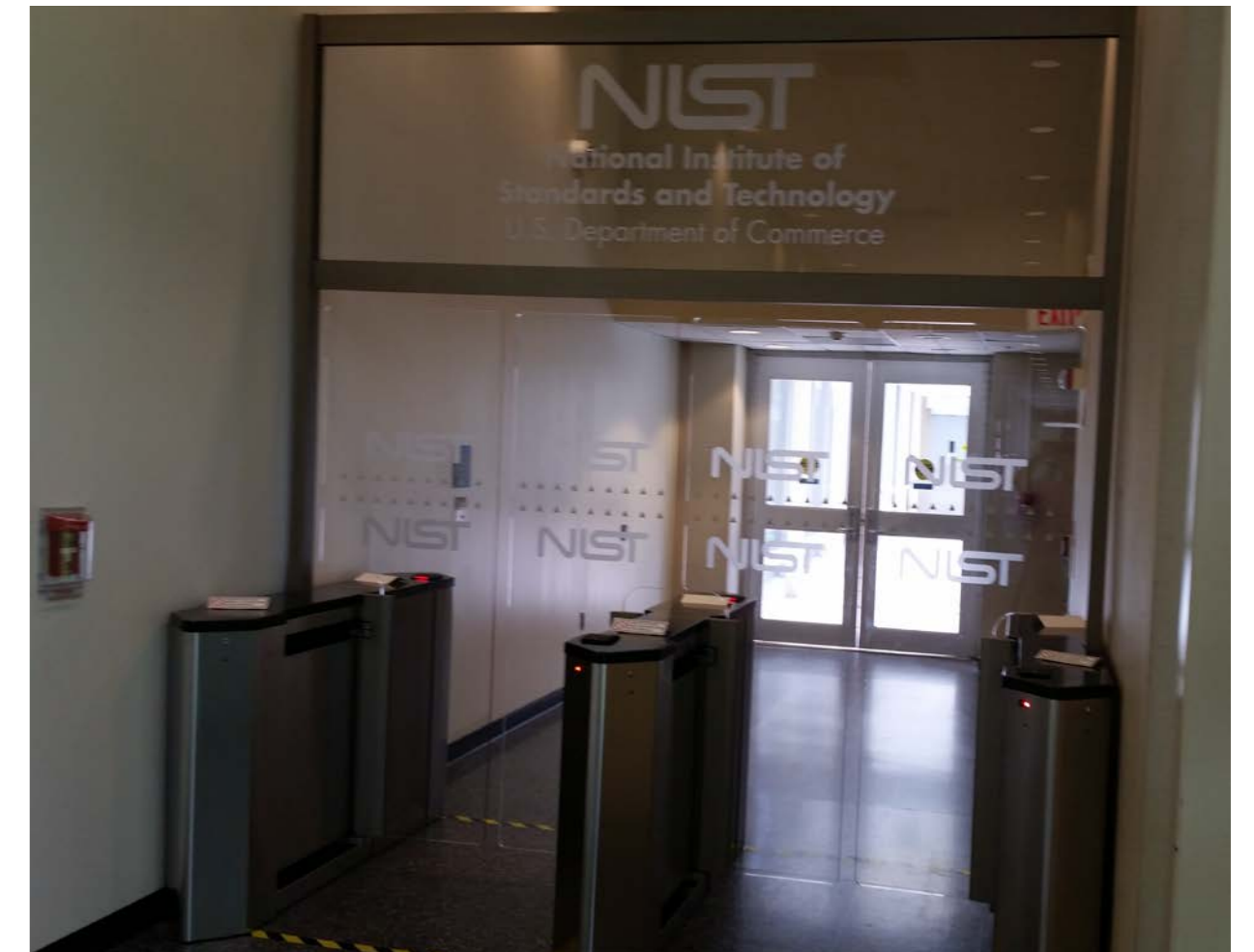
Security Turnstiles for access control to lab buildings adjacent to Bldg. 101 in Gaithersburg
