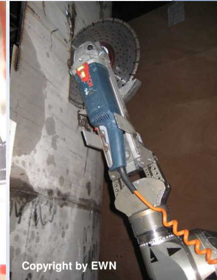
Cutting 10 mm thick tank wall
