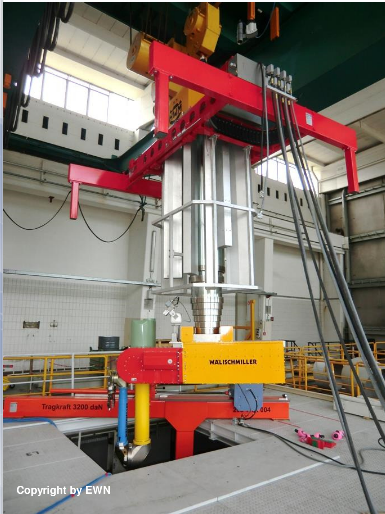
Verifying of Vertical Access conditions
