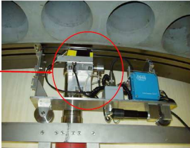
Single Device for Inspection and Laserscan of seal groove surfaces at the RPV closure head
