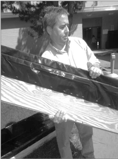
Exhibit 13. Showing how to hold a chute for the pour.
