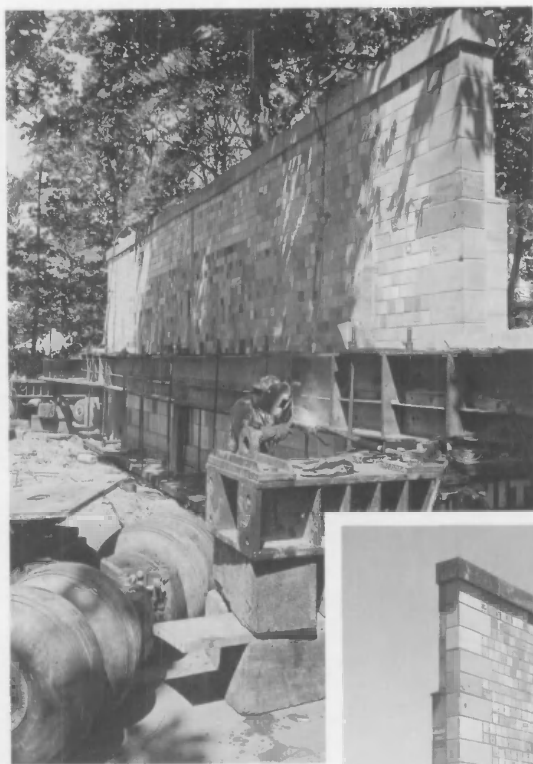
Left: A workman welds the framework of the apparatus that will carry the test exposure wall from the old site to Gaithersburg.
