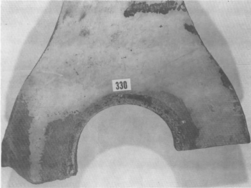
Figure 1: Inboard piece of the broken eye from the Point Pleasant Bridge. The north face is shown, and the lower side of the eye is at right.
