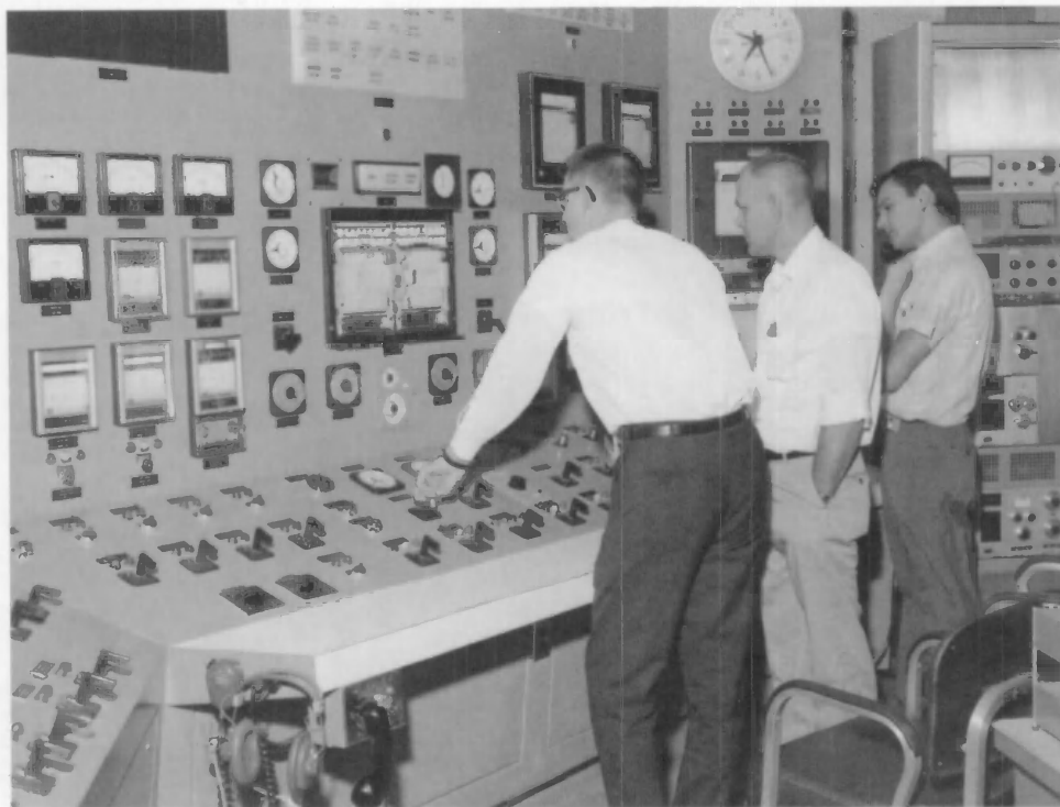
Change in the neutron flux in the NBS Reactor was monitored in the control room by (from left to right) Larry Smith, Arthur Chapman, and Albert W. Crebs as control rods were withdrawn to achieve criticality.
