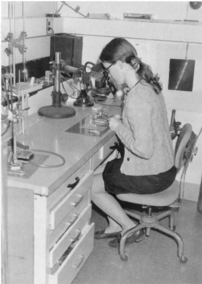
Sharill Wood welded platinum wires to fabricate a platinum resistance thermometer intended for use at temperatures as high as 1100 °C.
