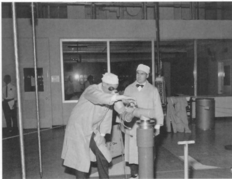
During the fueling process prior to criticality tests, Harry H. Landon, Chief of the NBS Neutron Nuclear Physics Section, checked the nuclear reactor core configuration through a periscope while Robert S. Carter, Chief of the Neutron Solid State Physics Section, observed.
