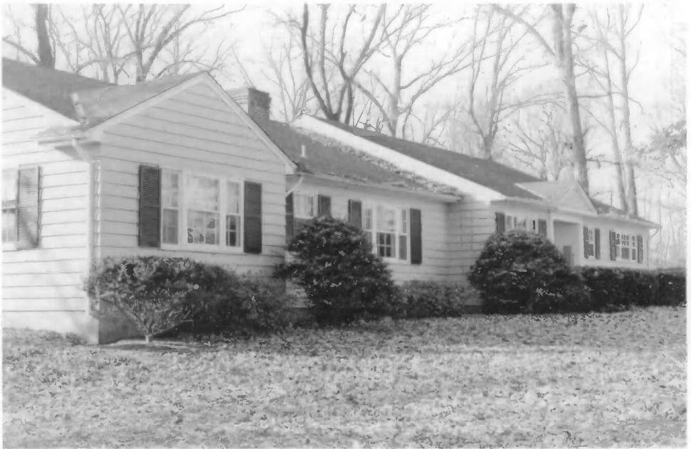
The Bowman House, purchased from its former owners when NBS obtained the surrounding property for the Gaithersburg site, was used by the Building Research Division until it was converted into a day care center in 1983.
