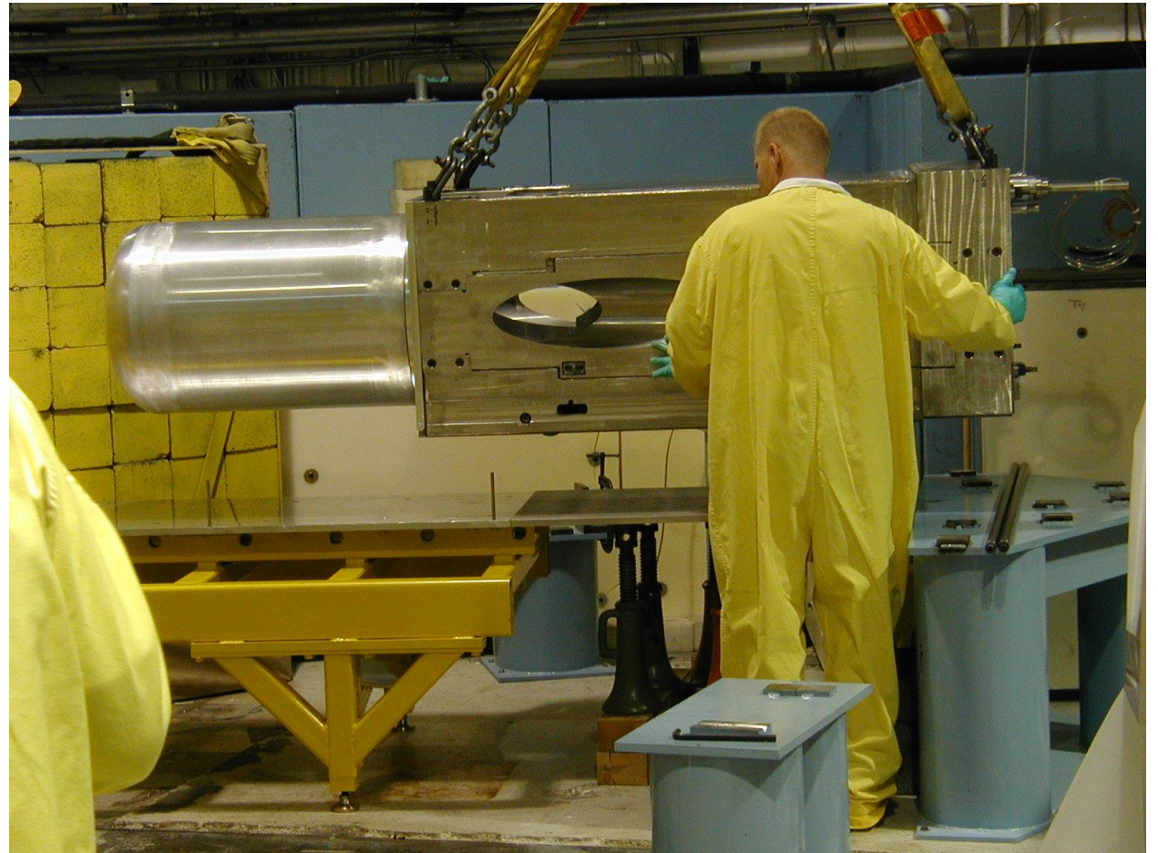
Installation of LH_2 CNS (Nov. 2001)
