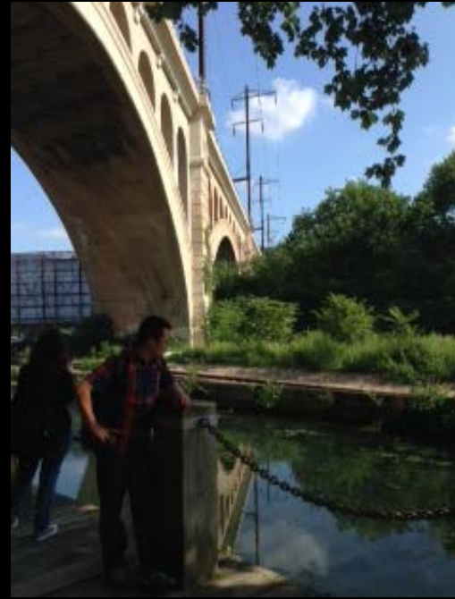
1918 Manayunk Bridge, Philadelphia, PA
