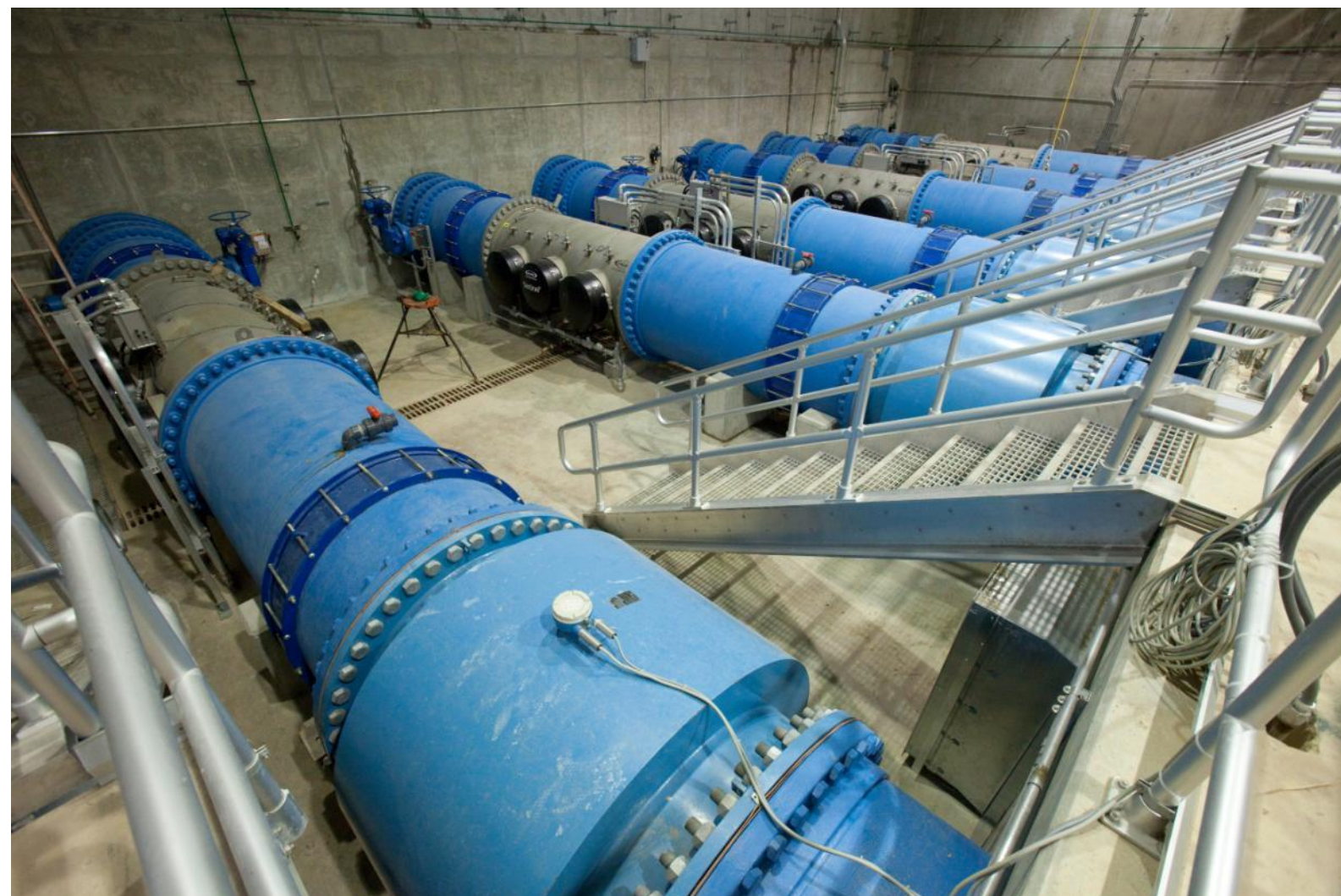
From ACE2011 UV Disinfection for the Real World: Back to Basics - WSSC Potomac Water Filtration Plant, Brian Balchunas, - Atkins and Joe Johnson - WSSC
