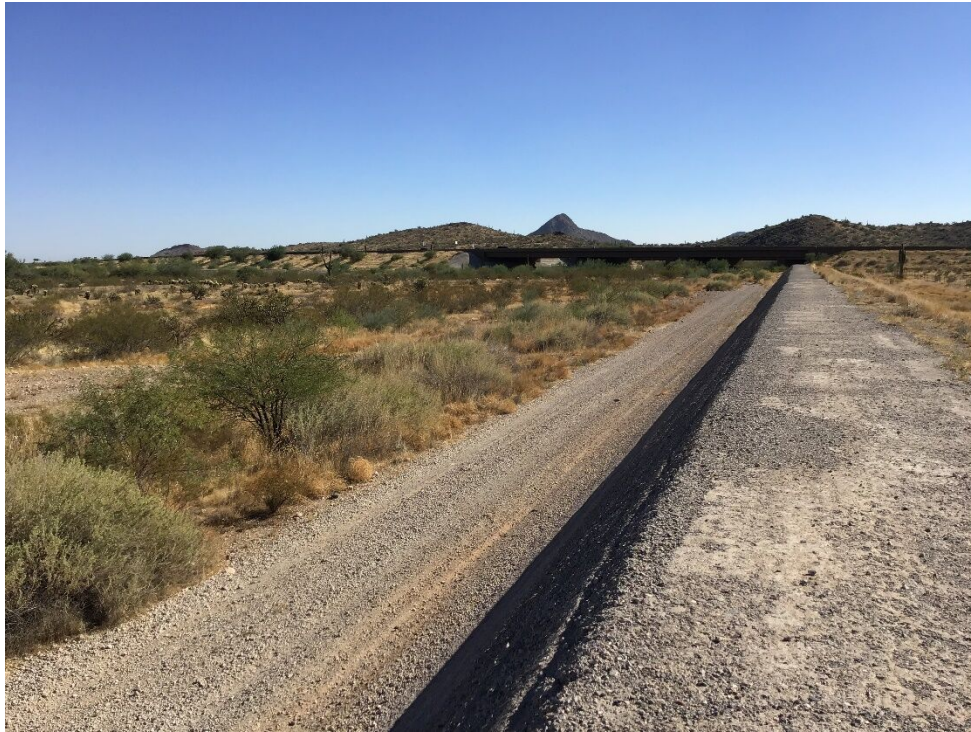
Photo 31 - View of Deadman Wash and Arizona State Route 303 from berm to northwest, facing south.
