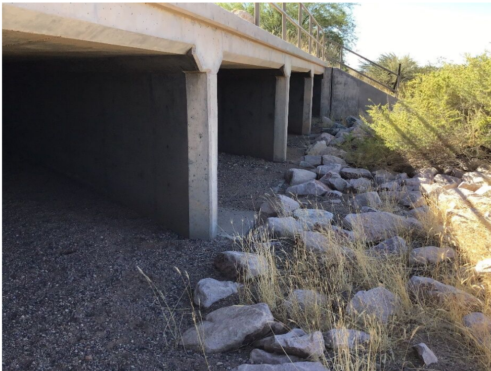
Photo 40 - View of culvert at southeast corner of PSB.
