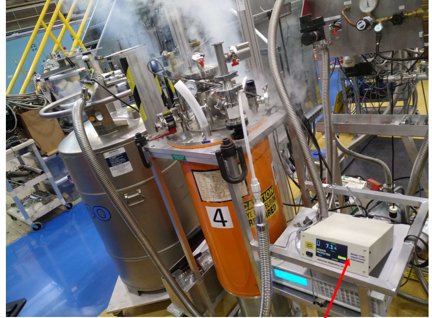
Cryogen level controller
