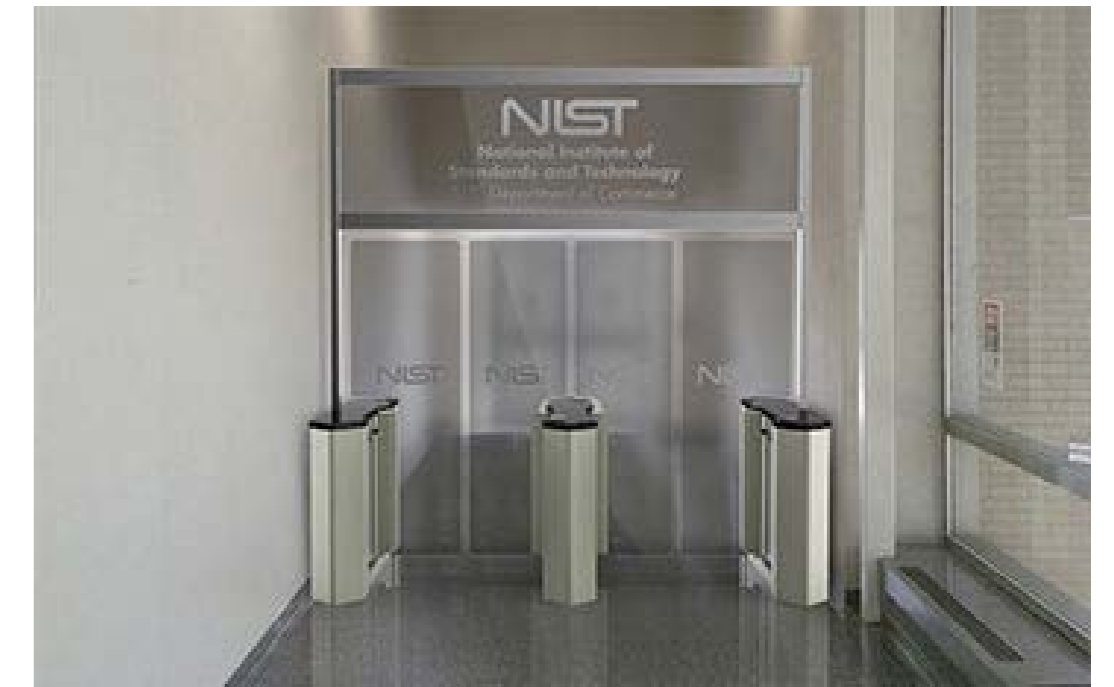
Artist drawing of Security Turnstiles for access control to lab buildings adjacent to bldg. 101
