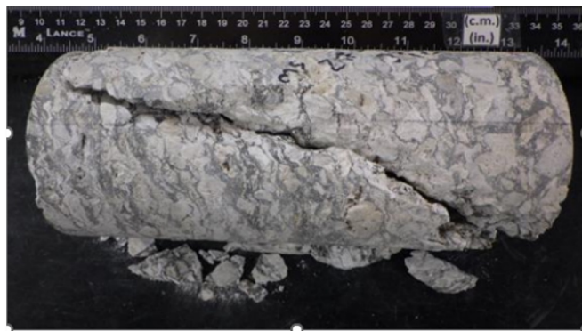
Example foundation pile-shaft core with a low compressive strength test result.
