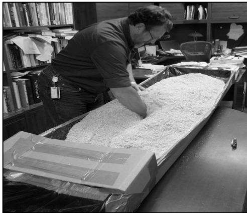
Figure 3-18. Spreading Bedding Material
